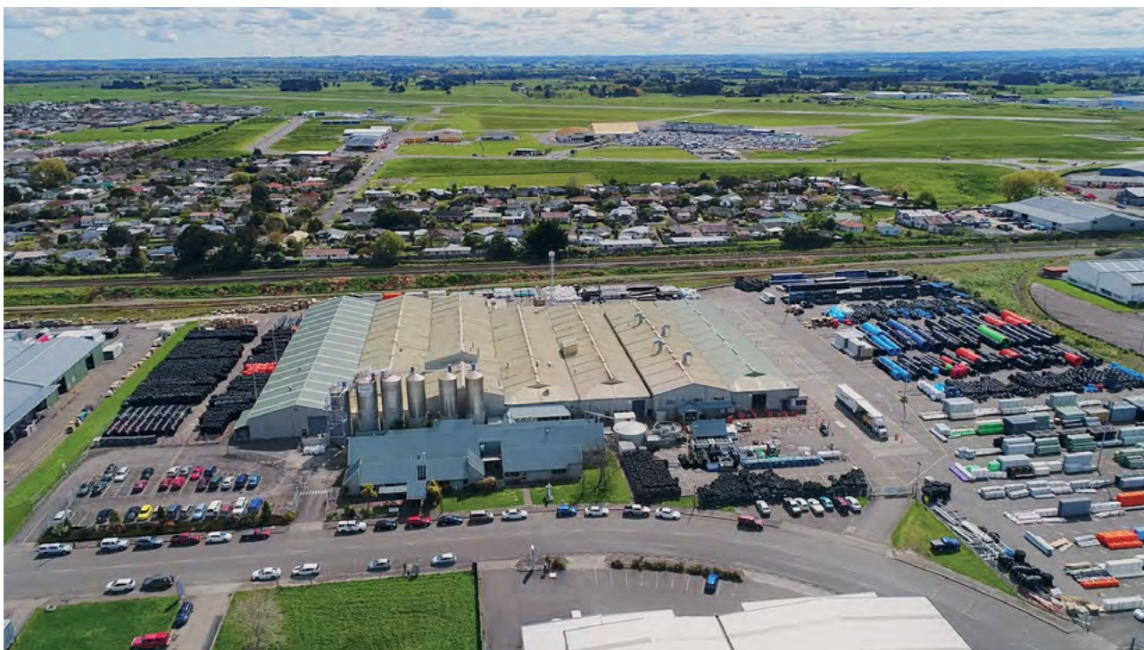
Iplex® Pipelines manufacturing plant and distribution hub in Palmerston North, New Zealand.
