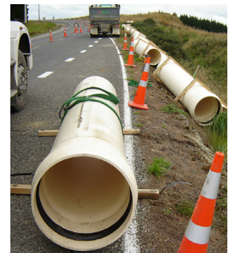
DN575 (630mm OD) PN9 WHITE RHINO for a wastewater outfall, installed under a sealed road, Edendale, Southland.
