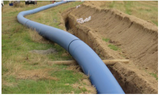
Aokautere falling water main
