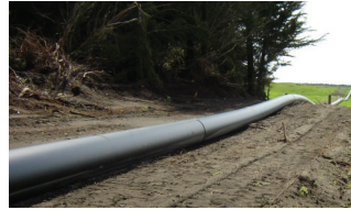
Waitara to New Plymouth wastewater rising main
