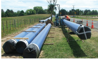
Papamoa trunk water main
