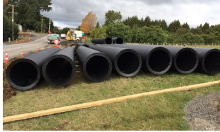
Tauranga Sewer transmission main
