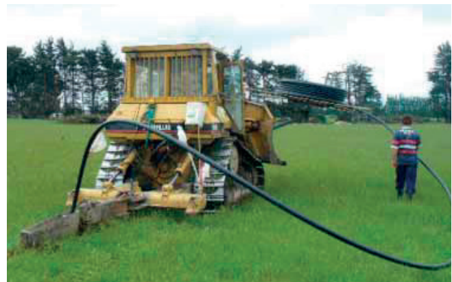
Installation of Blackline™ pipe by mole plough
