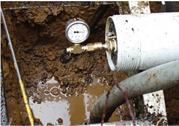
Figure 9.0 Field Testing, DN150 Restrain™ Sewer Pipe.
