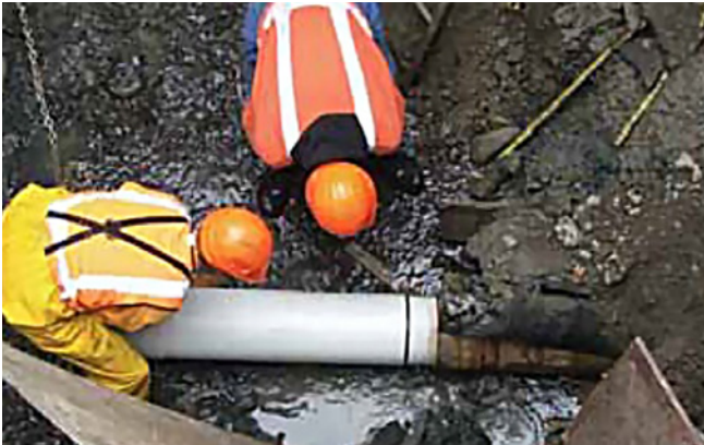
Figure 8.8 Typical Static Hydraulic Pipe Bursting installation DN225 x 3m Restrain™ Sewer Pipe.
