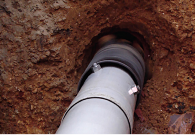
Figure 8.7 Typical reaming or pipe eating using a traditional Horizontal directional drill.
