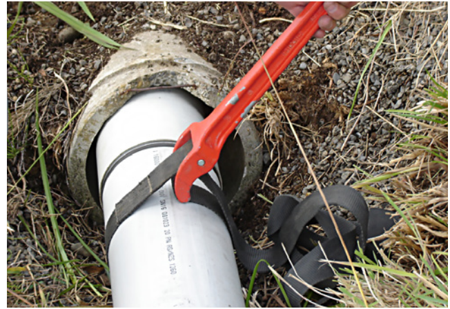
Figure 8.21 Assembling Restrain™ joint with strap wrench
