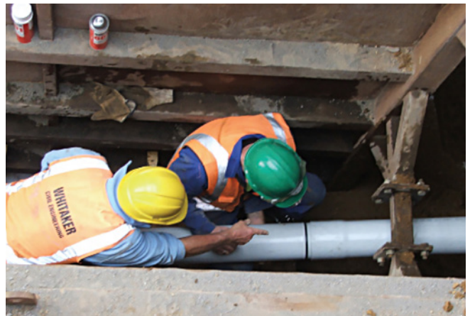
Figure 8.4 Typical HDD cartridge style pull-back between trench shields at a depth of 4.5m. DN150 x 6m Restrain™.
