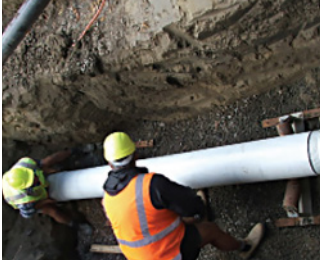
Figure 8.12 Installation Pit.
