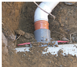
Figure 8.6 Restrain™ Quick Fit Saddle.
