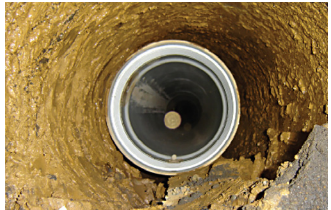
Figure 8.19 PTMT using DN225 x 2m Restrain™ Sewer Pipe. Installed at 0.04% grade.
