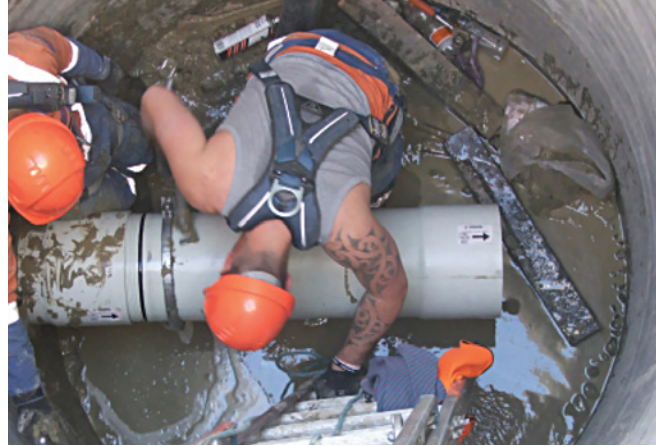
Figure 8.2 Typical HDD cartridge style pull-back within a 1.8m diameter x 4.5m deep manhole structure installing DN300 x 1m Restrain™ Sewer Pipe.
