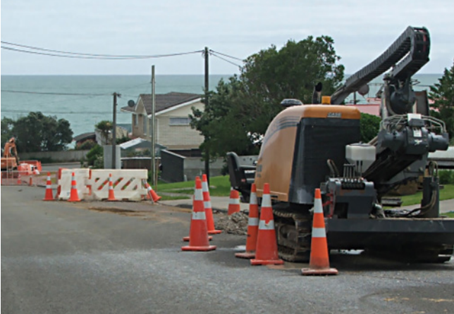
Figure 8.1 Typical cartridge style HDD pull-back.
