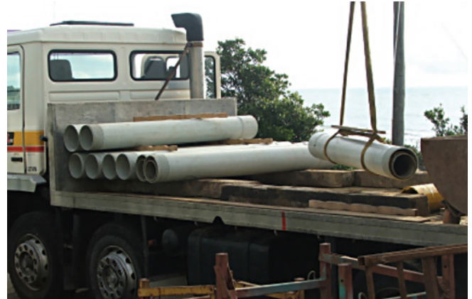
Figure 8.18 PTMT, DN225 x 2m Restrain™ Sewer Pipe, with auger section inserted.
