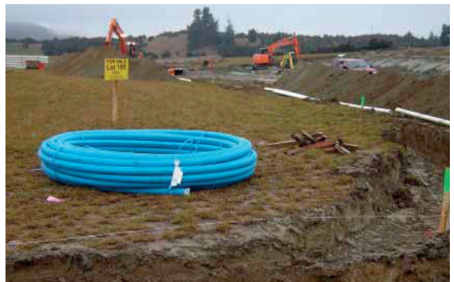
Coil of DN 63 PN 12.5 BlueLine polyethylene pipe on site, near Lake Wanaka.
