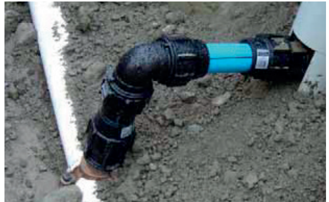
BlueLine pipe and Plasson Line 7 compression fittings used for a water service connection off a PVC-O main to a residential property near Wanaka.
