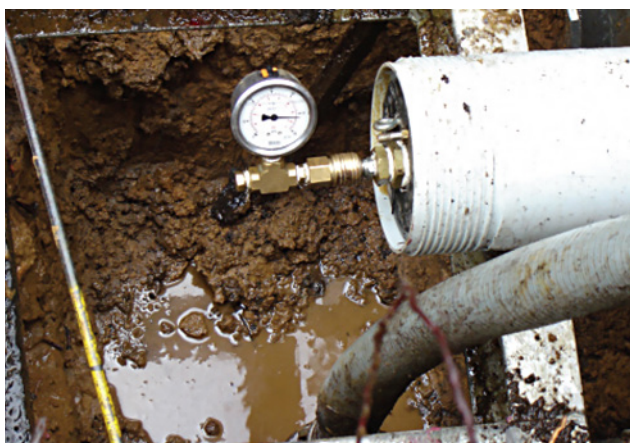
Figure 9.0 Field Testing, DN150 Restrain™ Sewer Pipe.
