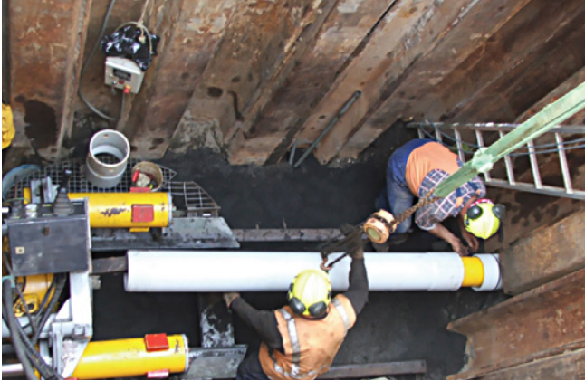
Figure 8.17 Typical Micro Tunnelling installation.
