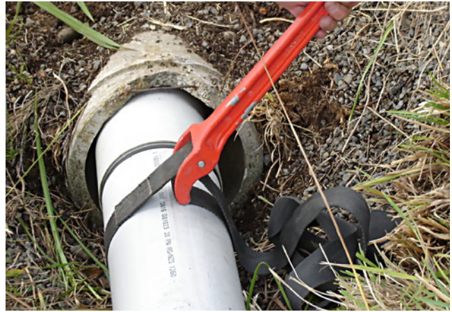
Figure 8.21 Assembling Restrain™ joint with strap wrench
