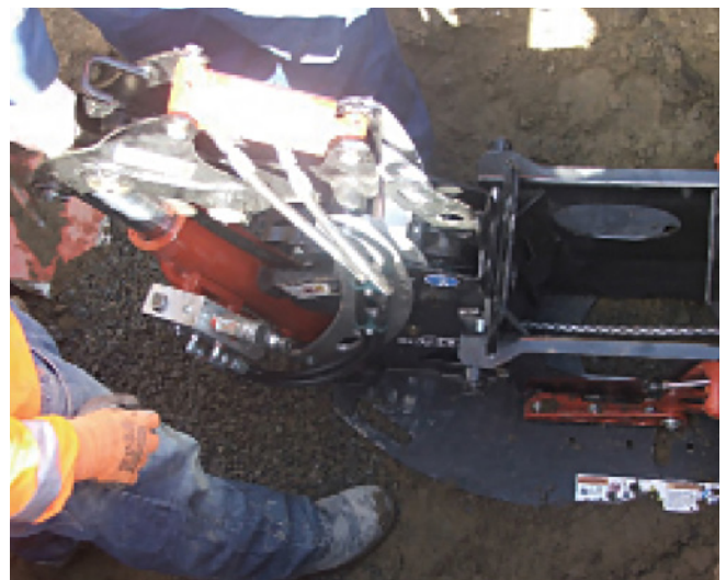
Figure 8.15 Receiving Pit with Hammer Head PB 30 Static pipe bursting unit.
