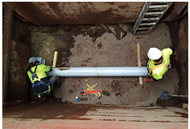
Figure 8.3 Typical HDD cartridge style pull-back within trench shields, 7m deep. DN225 x 3m Restrain™.
