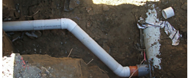
Figure 8.16 Restrain™ Sewer, Lateral Pipe & Quick Fit Saddle installed.
