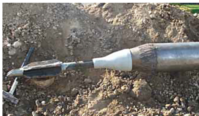
Figure 8.10 Typical External "Cone Style" Bursting Head. Upsize of existing 100mm CI pipe with new PVC pipe.
