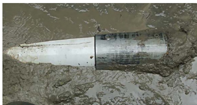
Figure 7.4 Typical free flowing drill mud/lubricant.
