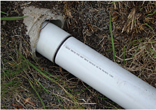
Figure 8.20 Typical Slip Lining installation using DN150 x 6m Restrain™ Sewer Pipe.
