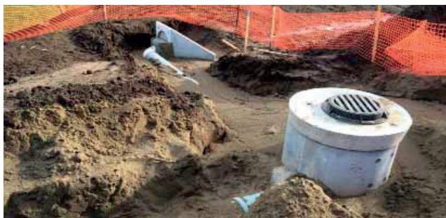
DN300 SN4 SUPERSTORM™ road sump lead pipe, and discharge pipe to wing wall. SH1 McKays to Peka Peka Expressway, Kapiti Coast.
