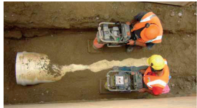
DN600 PVC-U stormwater pipe, showing a deep installation with correct mechanical side compaction of bedding and surround materials in layers, Edendale, Southland.
