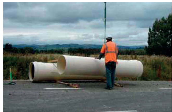
DN600 PVC-U stormwater pipe, showing correct lifting with nylon strap and dunnage protection under pipes on the road. Edendale, Southland.
