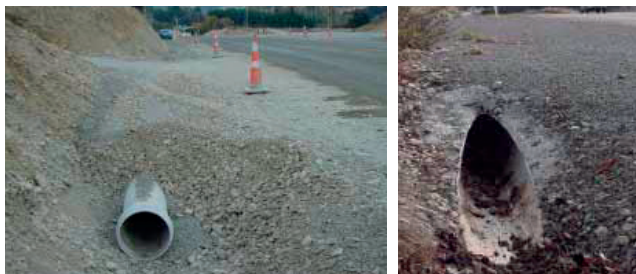
DN300 PVC-U stormwater pipe used as a road access culvert. (Left) Immediately after installation and (right) 4 years later, showing the effectiveness of well placed and thoroughly compacted bedding and surround aggregate material, SH1, Waianakarua, near Oamaru.
