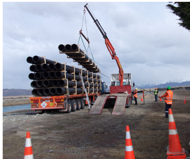
DN500 PN8, PE100 pressure water main pipe lengths in factory transport crates, being unloaded on site, Lake Tekapo Canal, Mackenzie District
