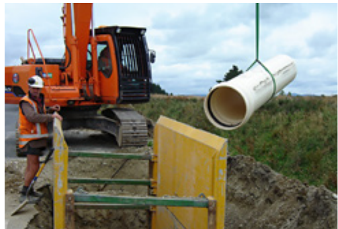
Installation of 3 metre lengths DN600 PVC-U stormwater pipe in trench shields, showing correct lifting with a nylon strop, Edendale, Southland.
