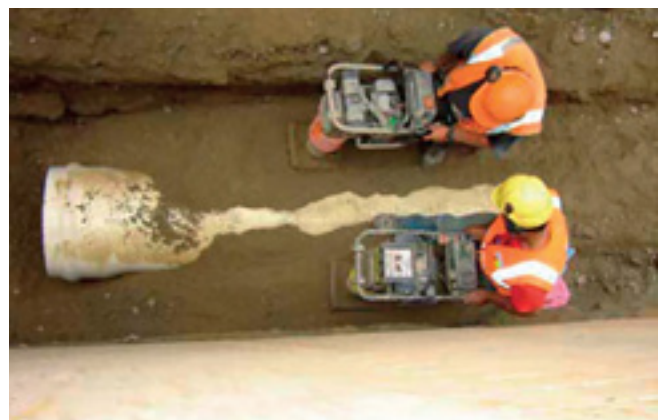
DN600 PVC-U stormwater pipe, showing a deep installation with correct mechanical side compaction of bedding and surround materials in layers, Edendale, Southland.
