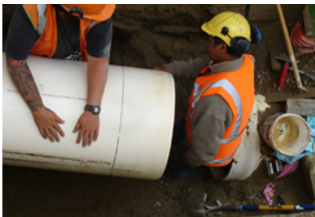
Preparing to join DN600 PVC-U stormwater pipe in trench, Edendale, Southland.
