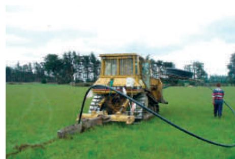
Mole Plough installation of Iplex PE pipes.
