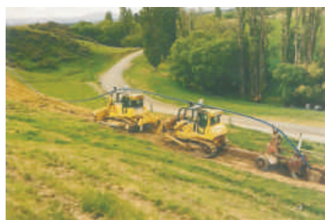
Mole Plough installation of Iplex PE pipes.
