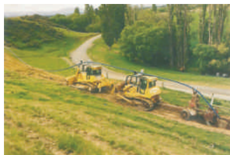
Mole Plough installation of Iplex PE pipes.
