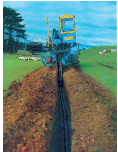
Installation of DN 110 NEXUSFLO subsoil drain by chain trenching, with laser control of gradient.
