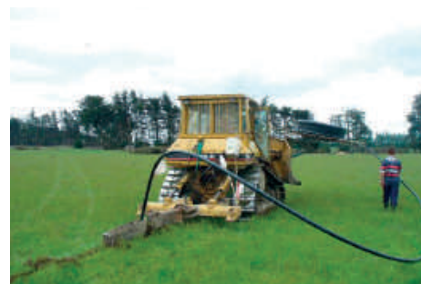
Mole Plough installation of Iplex PE pipes.
