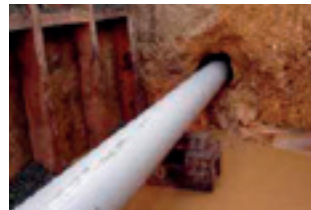
Assembly and installation of DN150 RESTRAIN™ gravity sewer, replacing an old EW sewer by pipe reaming with a horizontal directional drill, Invercargill City.
