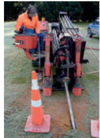
Assembly and installation of DN150 RESTRAIN™ gravity sewer, replacing an old EW sewer by pipe reaming with a horizontal directional drill, Invercargill City.
