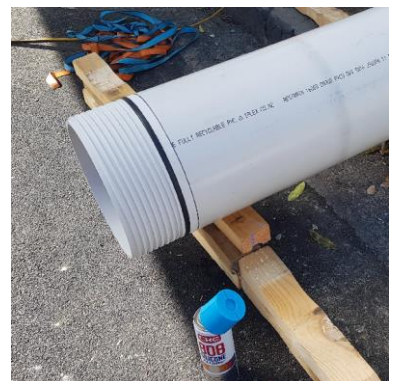
Approved Silicon Spray Lubricant Applied
