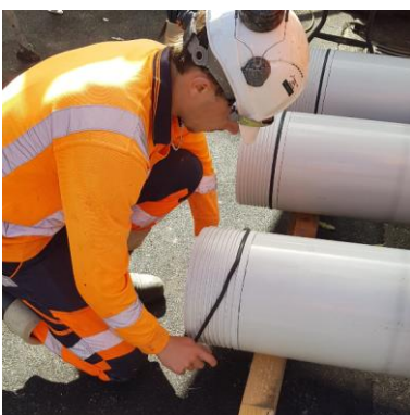
Fitting the Seal Ring
