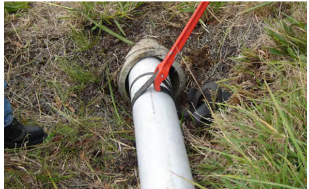
Figure 7.21 Assembling Restrain® joint with strap wrench
