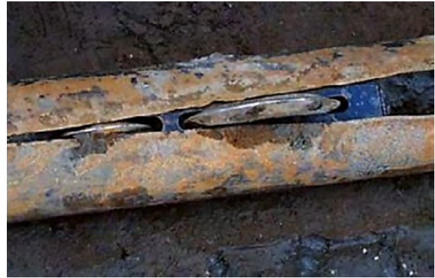
Figure 7.8 Typical "steel wheel" or "blade" type bursting heads.
