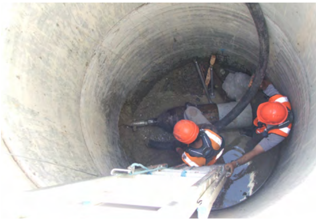
Figure 4.1 Restrain installation by Horizontal Directional Drilling
