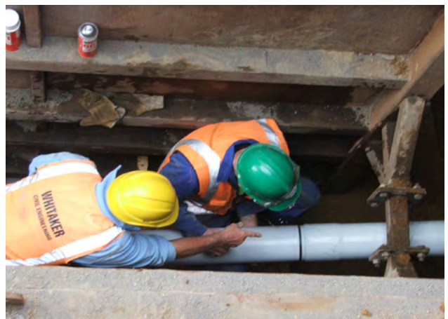
Figure 7.4 Typical HDD cartridge style pull-back between trench shields at a depth of 4.5m. DN150 x 3m Restrain®.
