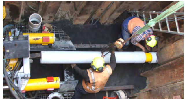
Figure 7.16 Typical Micro Tunnelling installation.
