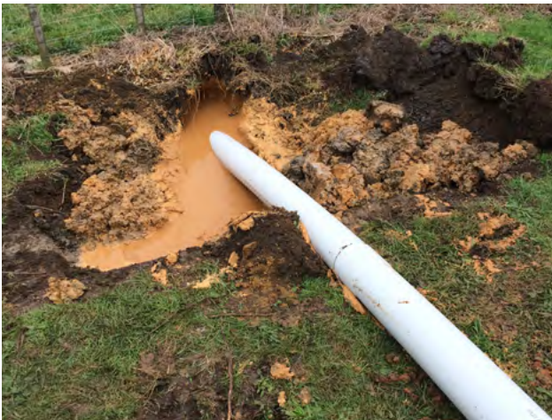
Figure 6.5 Typical free flowing drill mud/lubricant
