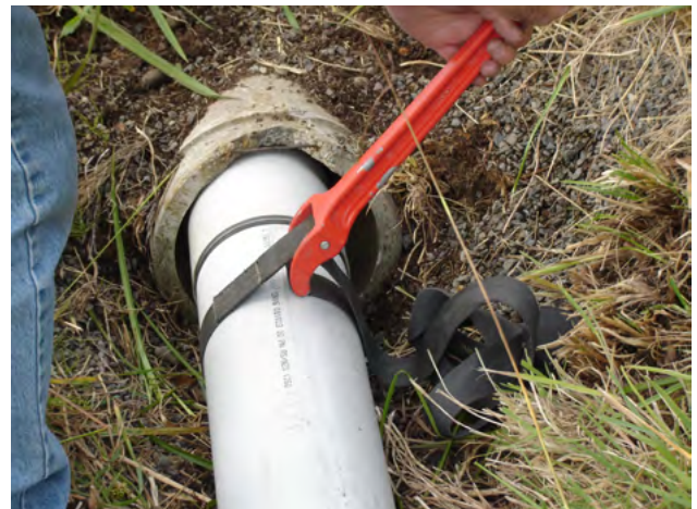
Figure 2.2 Restrain® installation by Slip lining into a concrete host
