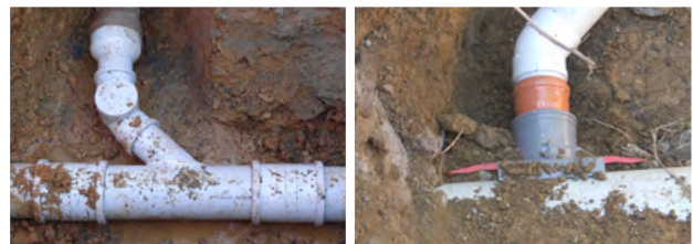
Figure 7.5 Plain ended wye junction. Figure 7.6 Restrain® Quick Fit Saddle.
