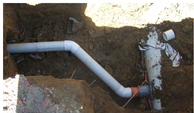
Figure 7.15 Restrain® Sewer, Lateral Pipe & Quick Fit Saddle installed
