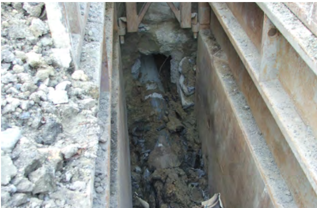
Figure 4.2 Restrain installation by Static Pipe Bursting of a concrete host
