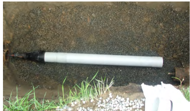
Figure 7.13 Pull Head with Restrain® Socket Starter Pipe attached
