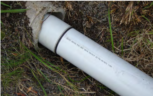
Figure 7.20 Typical Slip Lining installation using DN150 x 6m Restrain® Sewer Pipe, into a concrete Host.
