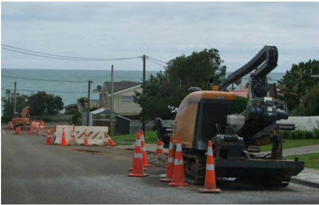
Figure 7.1 Typical cartridge style HDD pull-back.
