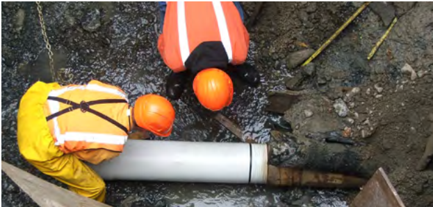
Figure 7.7 Typical Static Hydraulic Pipe Bursting installation DN225 x 3m Restrain® Sewer Pipe.
