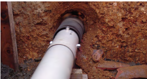
Figure 7.7 Reaming or pipe eating using a traditional Horizontal directional drill, applied to a glazed earthenware Host.
