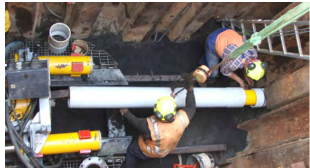
Figure 7.16 Typical Micro Tunnelling installation.
