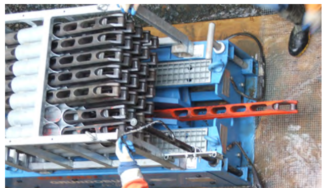
Figure 7.14 Receiving Pit with Hammer Head PB 30 Static pipe bursting unit.
