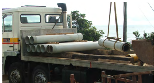
Figure 7.17 PTMT, DN225 x 2m Restrain® Sewer, Pipes with auger sections inserted.
