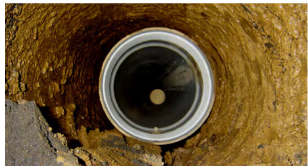
Figure 7.18 PTMT using DN225 x 2m Restrain® Sewer Pipe. Installed at 0.04% grade.
