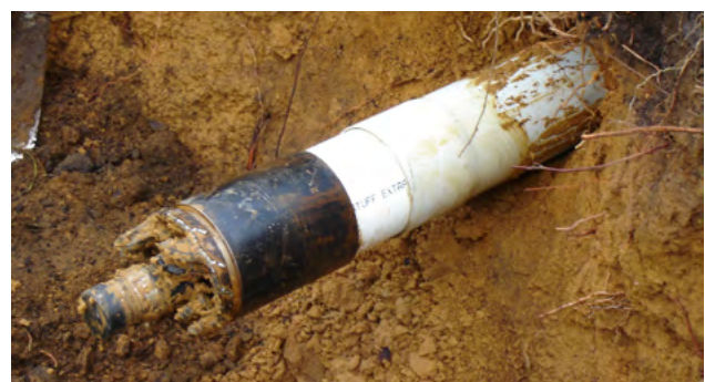
Figure 7.19 Lead auger with Restrain short starter pipe attached
