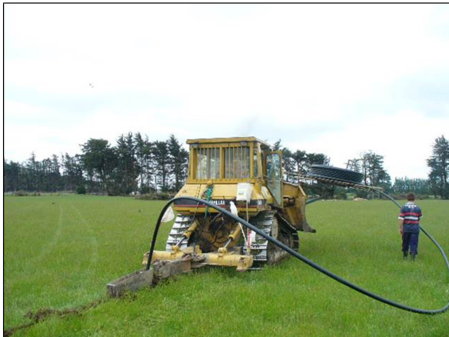
Installation of Iplex Redline pipe, using a Mole Plough
