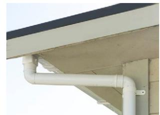
Support the offset by installing a pipe bracket directly below the lower offset bend.
