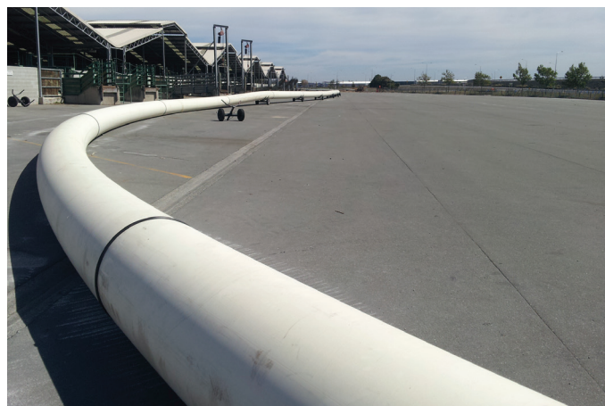
DN710, PN12.5, PE100 sewer rising main being prepared for installation by horizontal directional drilling. Pipe is black with a cream coloured jacket, identifying it visually as a pressure sewer in accordance with AS/NZS 4130.
