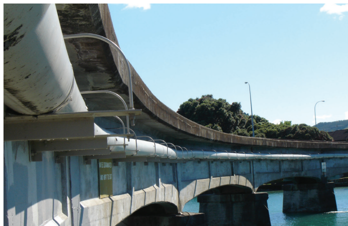
Support brackets for POLIplex pipe including allowance for expansion and contraction.
