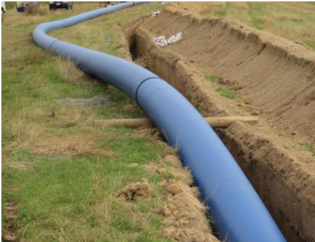
Aokautere falling water main
