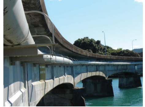
Gisborne wastewater rising main
