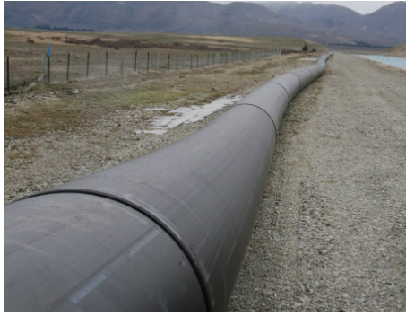
Tekapo diversion main
