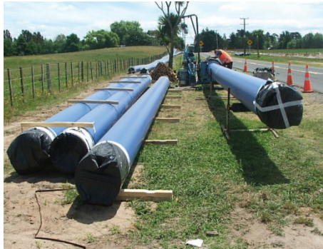
Papamoa trunk water main
