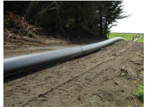
Waitara to New Plymouth wastewater rising main
