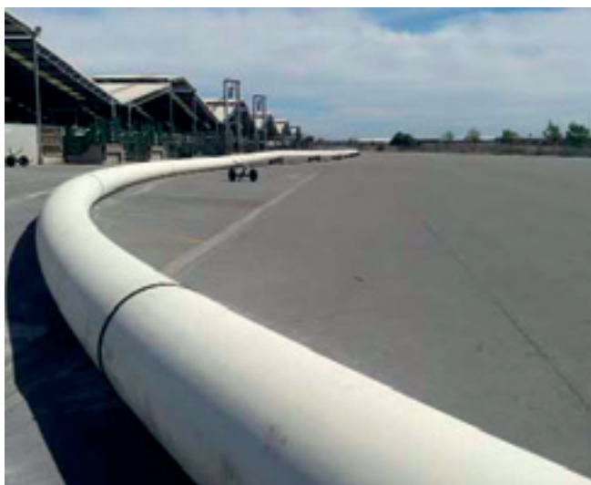
POLIplex DN710, PN12.5, PE100 sewer rising main being prepared for installation by horizontal directional drilling. Pipe is black with a cream coloured jacket, identifying it visually as a pressure sewer in accordance with AS/NZS 4130, Christchurch City.
