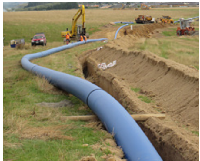
POLIplex DN 500 PN PE100 pressure pipe coloured black with blue jacket identifying it as a pressure water mains, Manawatu.
