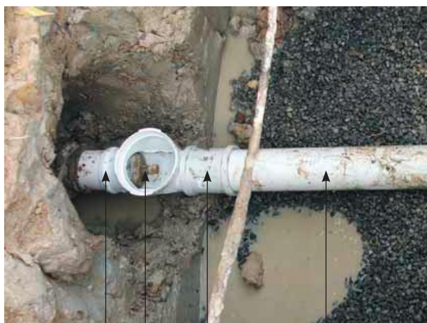
Figure 36 Typical positioning of hydrostatic test plug
