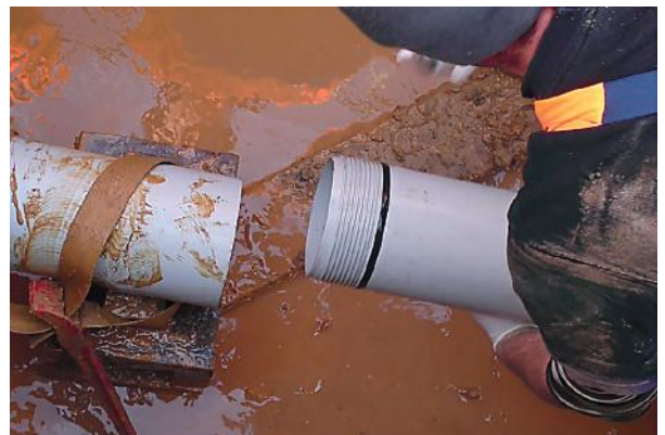
Restrain™ threaded spigot and socket pipe joint with axial end load restraint capability.
