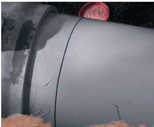
Figure 13 - Insert aligned lubricated spigot into socket
