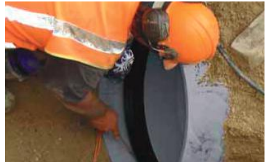
Figure 10 - Clean pipe seal within the socket
