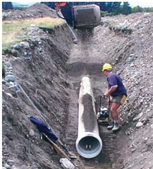
DN 450 Iplex PVC-U sewer rising main, laid near Te Anau in 2000, which has endured undamaged, all earthquakes in the Te Anau area, 2000 to 2019.
