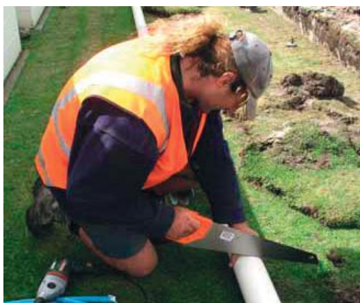
Figure 4 - Cutting pipe with hand saw
