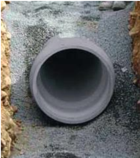
Figure 15 - Thoroughly clean and dry empty pipe socket
