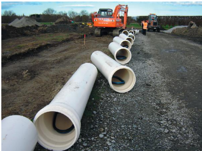
DN 450 Iplex PVC-U sewer rising main, laid near Belfast, Christchurch in 2005, which endured the 2010 and 2011 Canterbury earthquake sequences undamaged,
