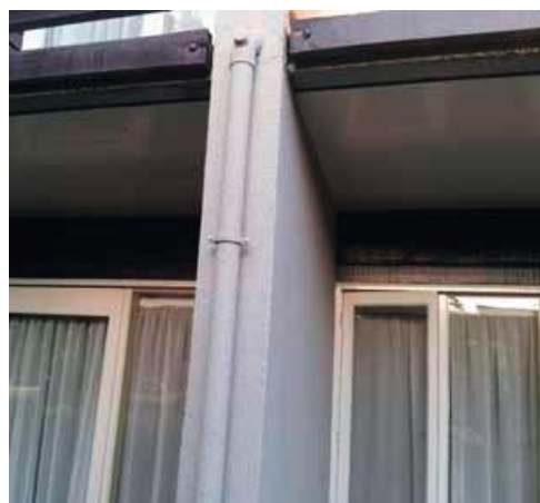
Figure 1: Exposed PVC pipe protected from weathering with UV resistant water-based paint, Dunedin City.
