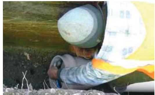
Figure 12 - Apply lubricant to seal with a brush
