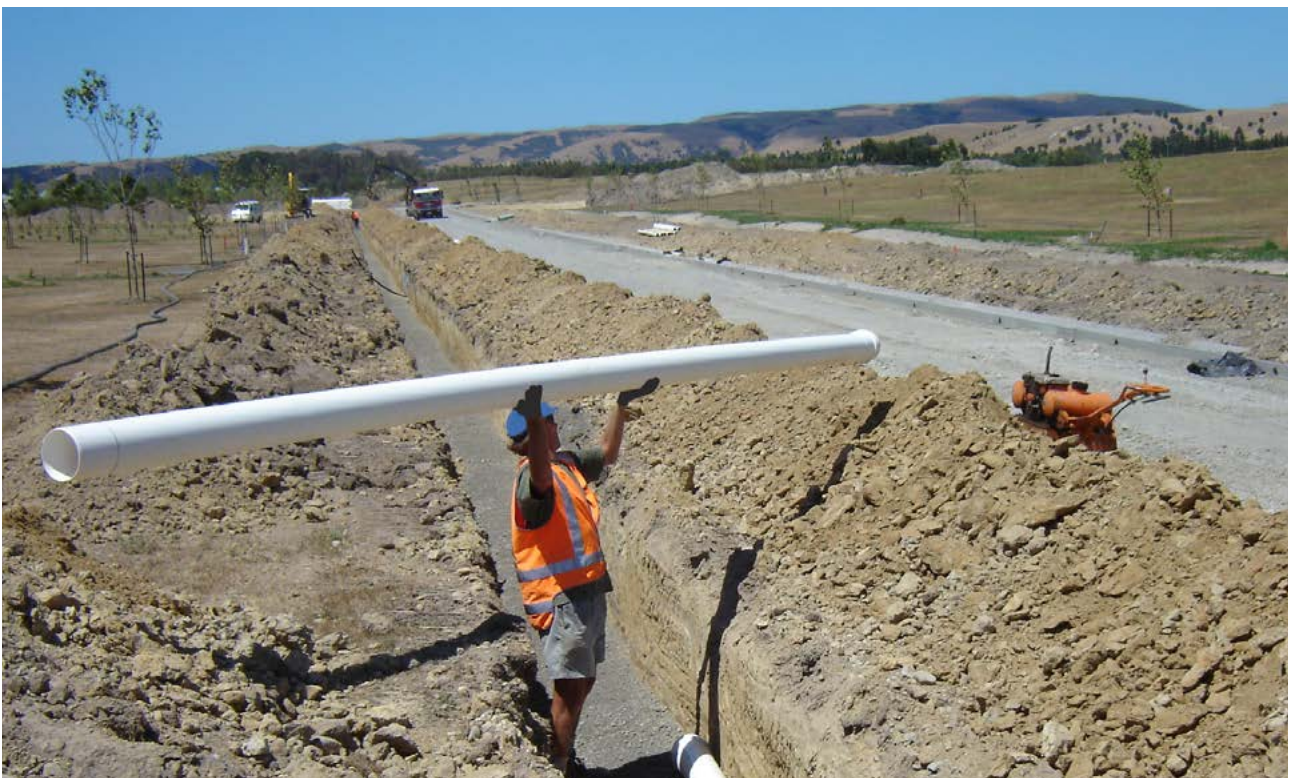
Iplex Apollo® PVC-O Series 1 pressure pipe used for water distribution, in a residential subdivision near Martinborough.
