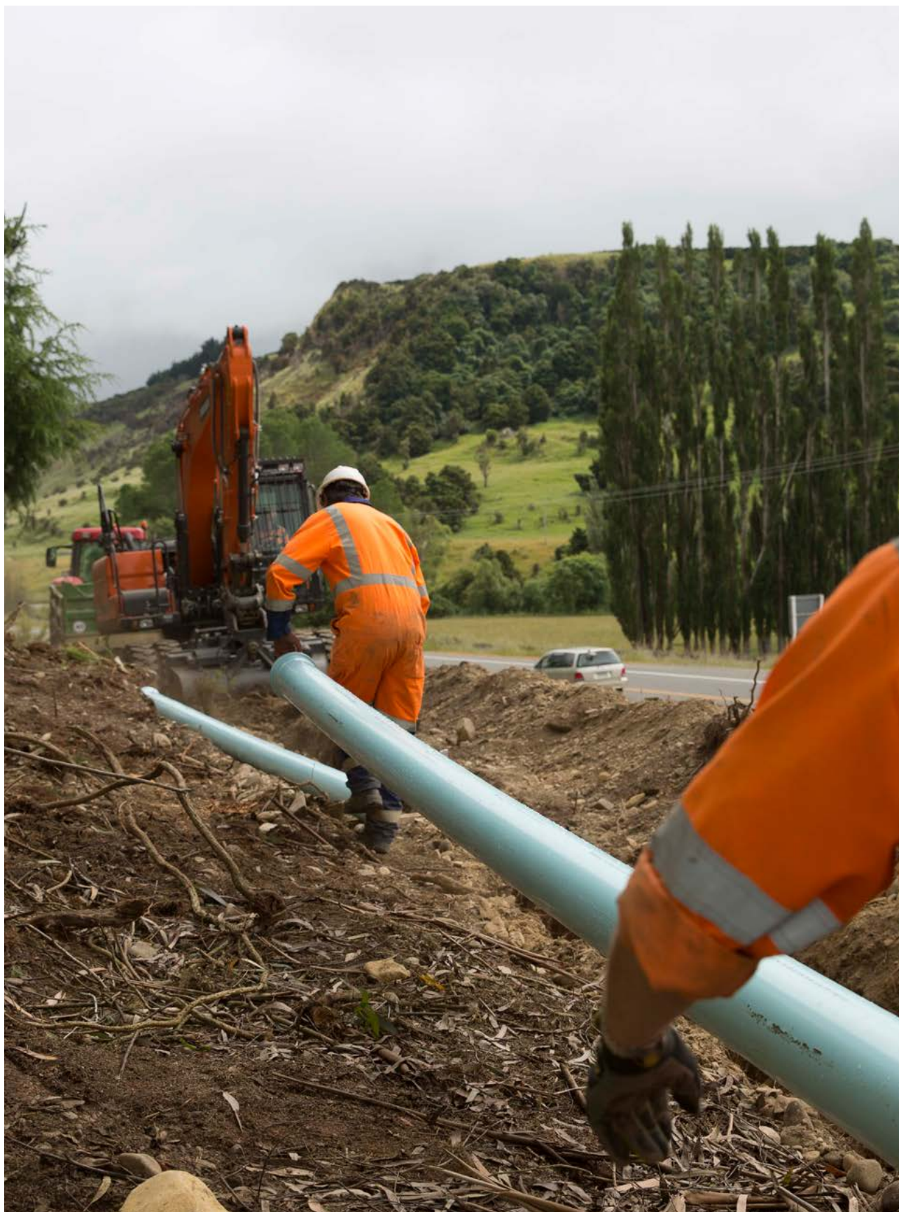
Iplex Apollo® Blue PVC-O Series 2 pressure pipe used in the Oamaru to Hampden water pipeline.
