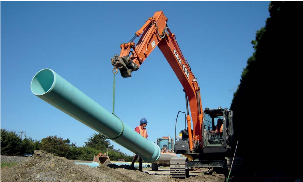
Iplex Series 2 PVC pressure pipe, used for a bulk transmission watermain, near Rangiora, Waimakariri District.
