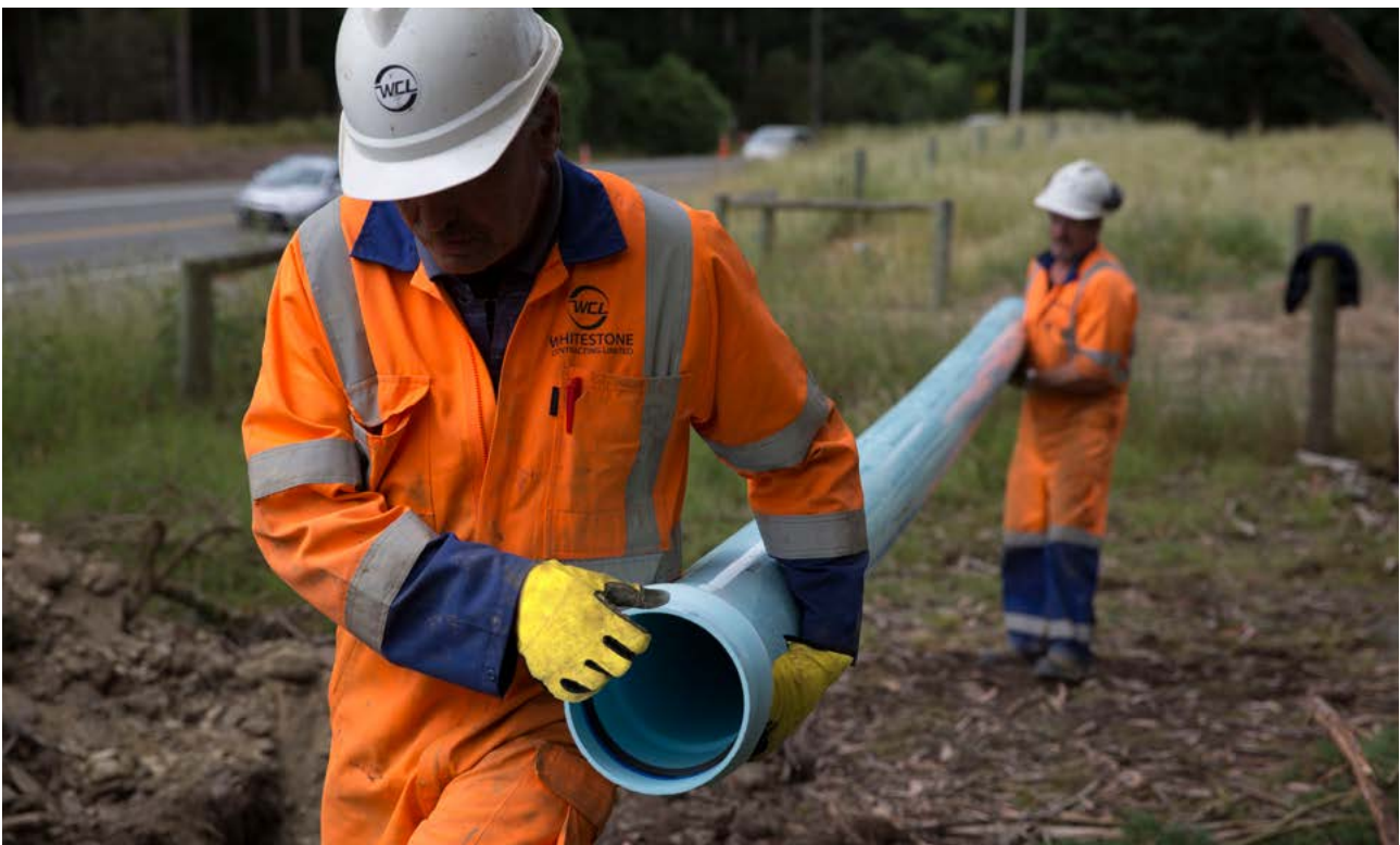
Iplex Apollo® Blue PVC-O Series 2 pressure pipe, used in the Oamaru to Hampden water pipeline.
