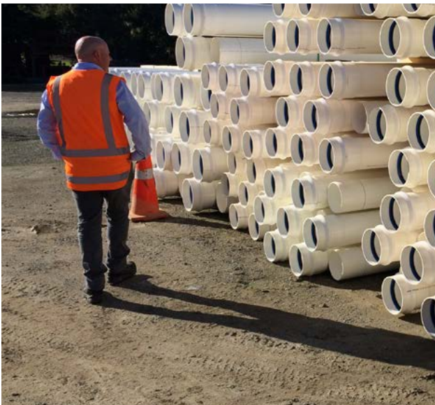
PVC pressure pipe showing storage on a project site.
