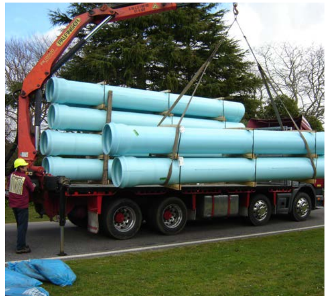
DN525 PVC pressure pipe showing “2 point support” lifting arrangement during offloading on a project site.
