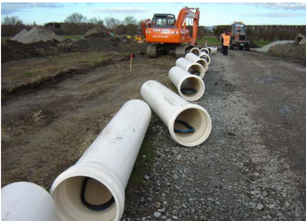
Iplex Novakey® DN450 PVC-U pressure sewer rising main, laid near Belfast, Christchurch in 2005, which endured the 2011 Canterbury earthquake sequences undamaged.
