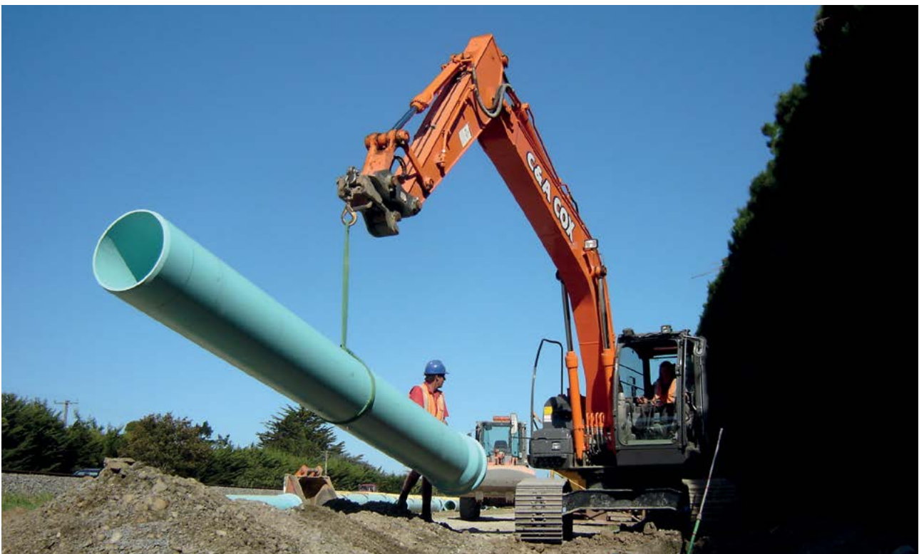
Iplex PVC Series 2 pressure pipe used for a bulk transmission watermain, near Rangiora, Waimakariri District.
