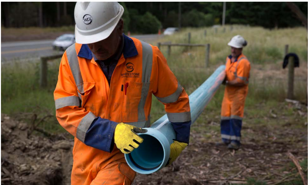
Iplex Apollo® Blue PVC-O Series 1 pressure pipe used on the Oamaru to Hampden Pipeline.
