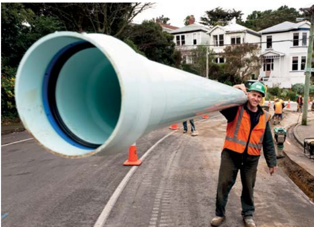
Iplex Apollo® Blue PVC-O DN150 PN16 pressure watermain, installed in Kelburn Parade, Wellington City, in 2011, specifically to improve seismic resilience in the area, which endured the November 2016 Kaikoura / Culverden earthquake sequence, undamaged.
