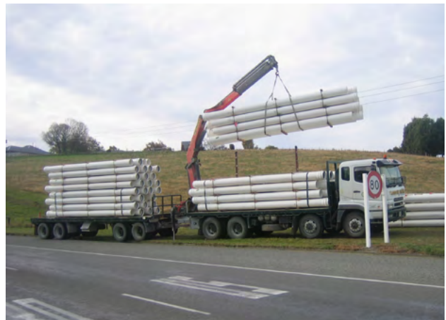
Figure 11.2 - Mechanical lifting, using two point suspension, and polymer slings, of DN 300 Series 1 PN 12.5 Iplex Apollo® PVC-O pipe in bulk crates, Timaru City
