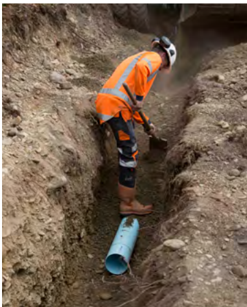
Figure 11.25 - Placing the selected size imported bedding aggregate, fully surrounding the pipe, Waitaki District
