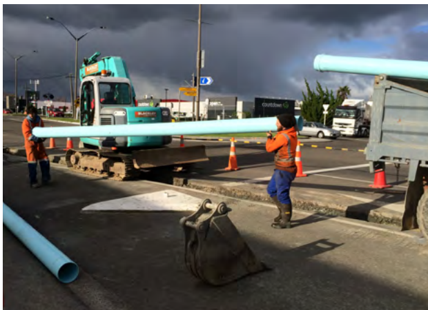
Figure 11.1 - Handling and unloading of DN150 PN 12.5 Iplex Apollo® PVC-O pipe, preventing abrasion damage from the truck deck or by impacting the road surface. - Feilding, Manawatu District
