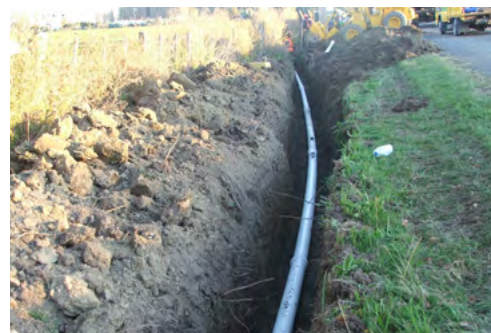
Figure 11.30 - DN 100 Iplex Apollo® PVC-O Series 1 PN 12.5 waste water transmission main, in 6m lengths, on a curved alignment, Gisborne District
