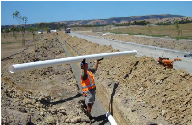
Figure 4.2 - Site handling and installation of Iplex Apollo® PVC-O DN 100 Series 1 PN 12.5, for water distribution in a residential subdivision near Martinborough
