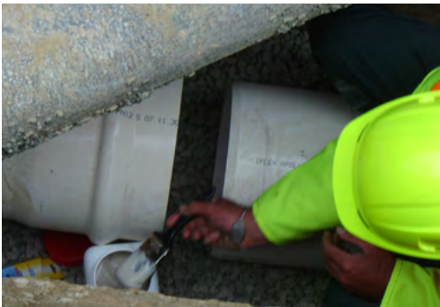
Figure 11.16 - Apply Medlube lubricant to both the seal and the spigot with a clean brush
