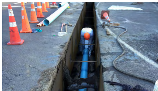
Figure 5.1 - Installing a DN 200 S2 PN 12.5 Iplex Apollo® PVC-O Water Main in a main highway crossing, through hydrocarbon- contaminated ground, Manawatu District
