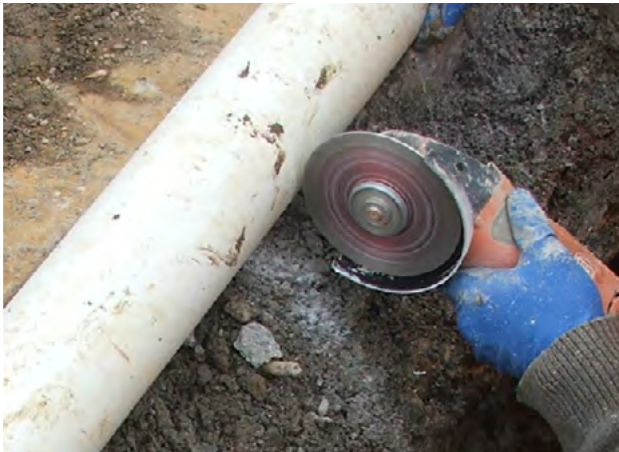
Figure 11.5 - Cutting pipe with power-driven masonry blade
