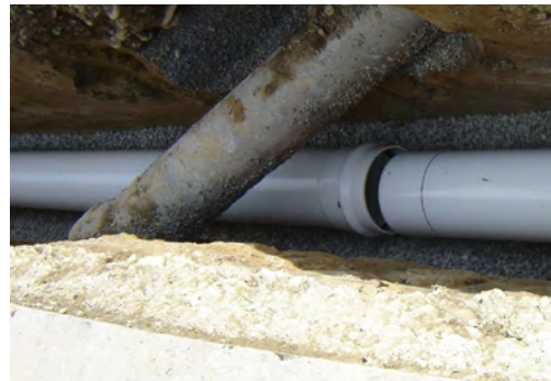
Figure 11.17 - Align the lubricated spigot with the socket mouth
