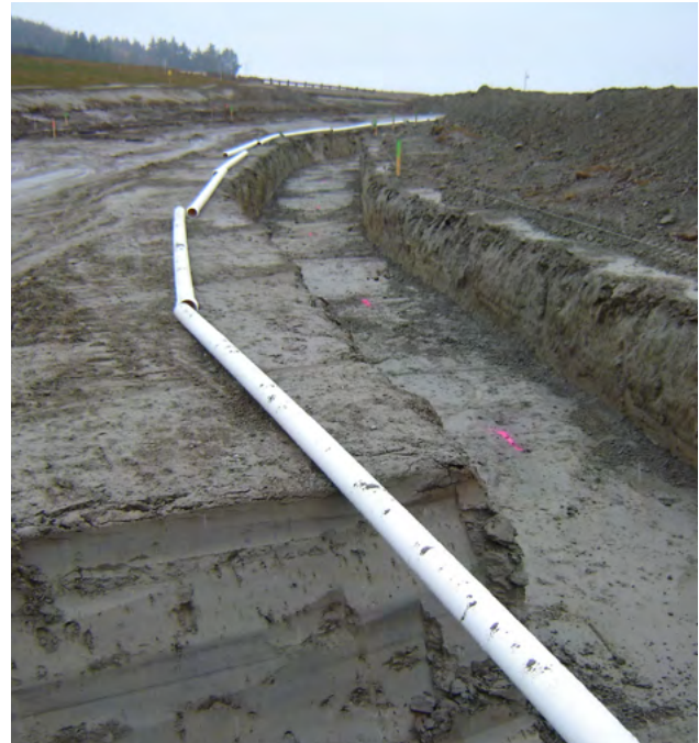
Figure 8.11 - Installing DN 100 S1 PN 12.5 Iplex Apollo® PVC-O pipes in sub-zero winter conditions, for a reticulation Water Main ,Wanaka, Queenstown Lakes District
