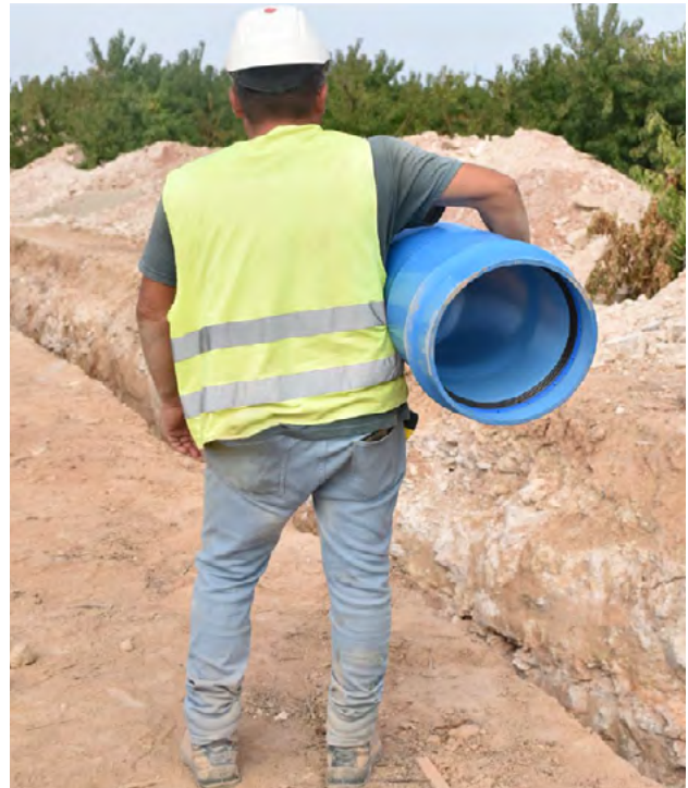
Figure 9.16 - Site handling Lightweight PVC-O DN 375 PN 16 22.5O Bend
