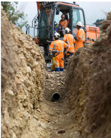
Figure 11.26 - Showing correct position of pipe, fully surrounded by selected size imported bedding aggregate, with all other larger size "as dug" aggregate, above the bedding, totally excluded from direct contact with the pipe, Waitaki District
