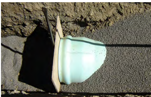
Figure 11.12 - Protect the clean socket from entry of dirt and grit, before joint assembly
