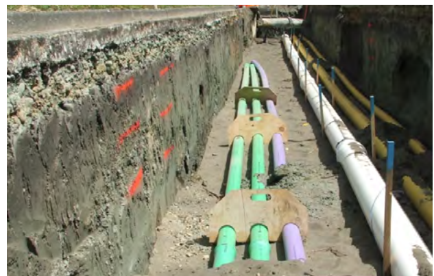
Figure 10.2 - Trench with temporary red index marks on the trench wall to guide backfilling and compaction in 300mm layers
