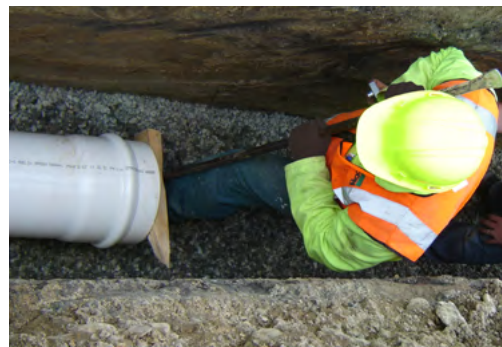
Figure 11.19 - Push pipe spigot into the socket through the seal ring using a bar, and wood block to protect the pipe end. DO NOT INSERT PAST THE WITNESS MARK
