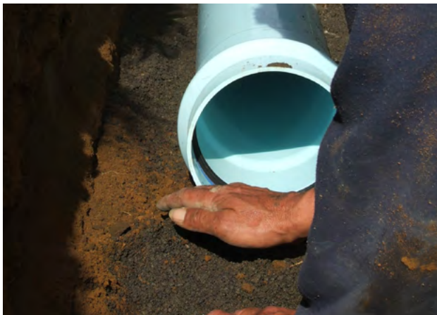
Figure 11.10 - Carefully clear away any dirt from the socket mouth
