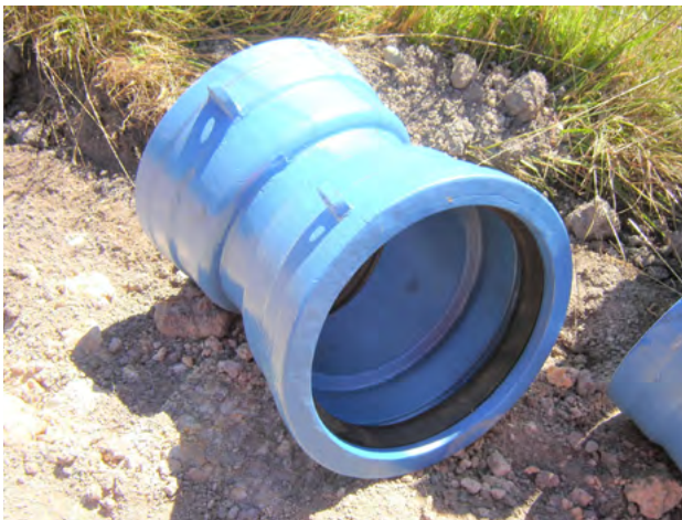
Figure 9.3 - Socketed Ductile Iron fittings should have a full circle pipe stop in the Socket, to butt the PVC pipe end against, when installing, to prevent over- insertion
