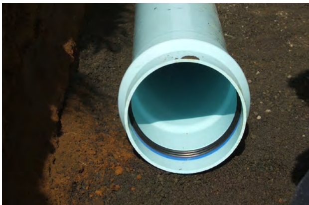
Figure 11.11 - Totally clean socket, ready for jointing
