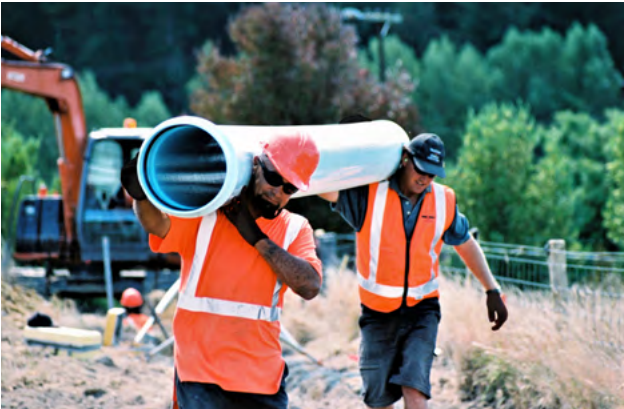
Figure 4.1 - Site handling of Iplex Apollo® PVC-O DN 250 Series 2 PN 12.5, for drinking water distribution, Nelson District
