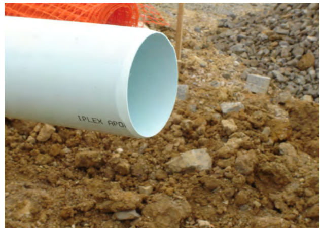
Figure 11.9 - Hand- chamfered Iplex Apollo® PVC-O pipe spigot
