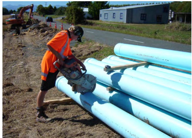
Figure 11.7 - Cutting pipe with power-driven masonry blade
