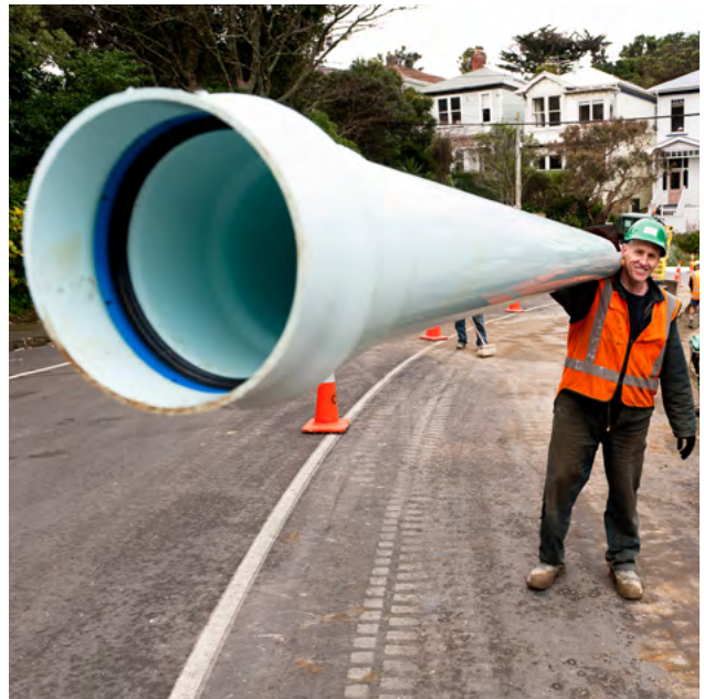
Figure 7.2 - Iplex Apollo Blue® PVC-O DN 150 PN 16 pressure watermain, installed in Kelburn Parade, Wellington City, in 2011, specifically to improve seismic resilience in the area, which endured the November 2016 Kaikoura/ Culverden Earthquake sequence, undamaged
