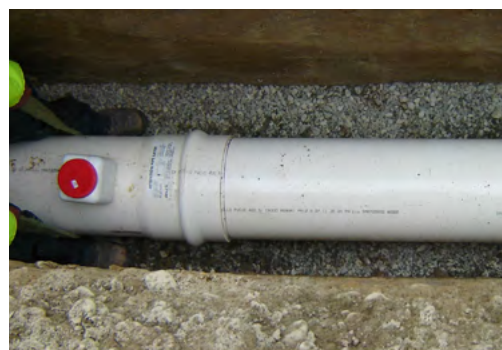
Figure 11.21 - Push joint home until witness mark remains just visible
