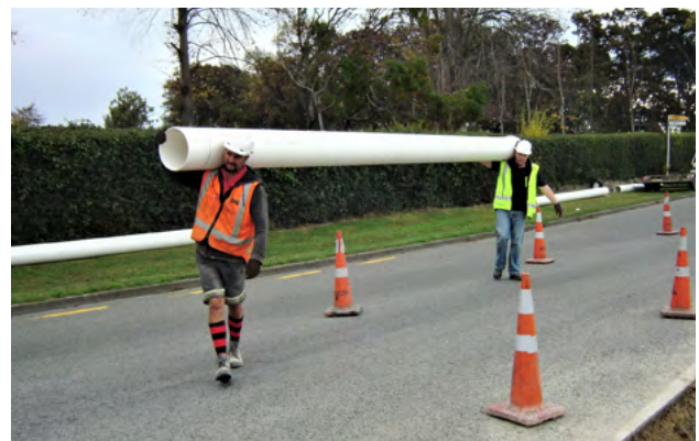
Figure 12.3 Site handling of Iplex Apollo® PVC-O DN300 S1 PN12.5 in 6m lengths, Timaru City
