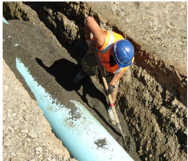
Figure 11.22 - Typical placement and "blinding": of granular bedding and surround material
