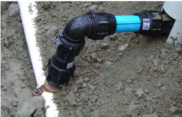
Figure 9.13 - Gunmetal tapping saddle with a Plasson "line 7" male threaded adapter, on white DN 100 Series 1 Iplex Apollo® PVC-O water main, connecting to a DN 50 Iplex BlueLine PE service lateral, and valve box, near Wanaka, Queenstown Lakes District
