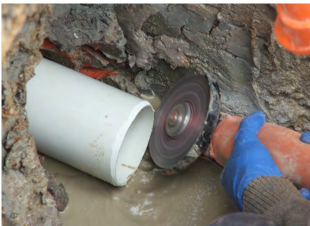
Figure 11.6 - Chamfering pipe with power-driven masonry blade
