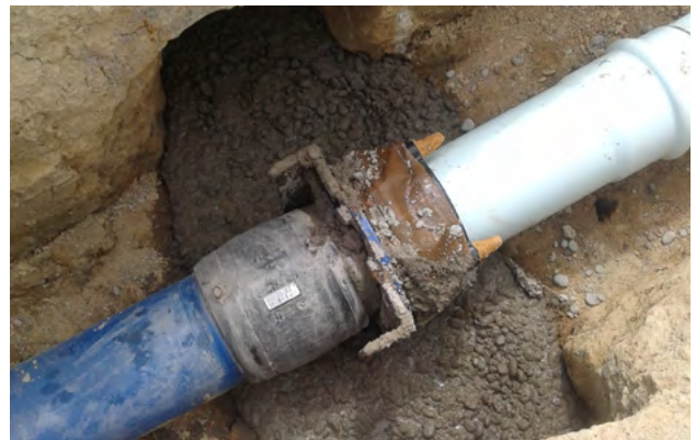
Figure 10.3 - Concrete thrust block with vertical tie bars, supporting an in-line flanged connection between Iplex Apollo® PVC-O and PE pressure pipe at a river crossing, Waitaki District
