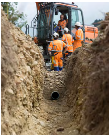
Figure 11.26 - Showing correct position of pipe, fully surrounded by selected size imported bedding aggregate, with all other larger size "as dug" aggregate, totally excluded from direct contact with the pipe, Waitaki District
