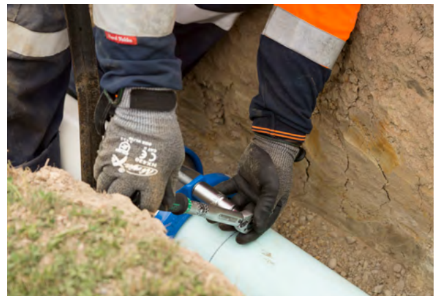
Figure 9.11 - Use of a torque wrench during final tightening of the bolts on an "AVK" brand Universal Coupling, installed on DN 100 Series 1 Iplex Apollo® PVC-O pressure pipe
