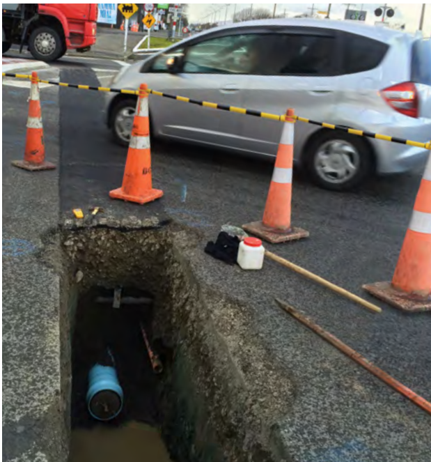
Figure 10.1 - Iplex Apollo® PVC-O, DN 150 S2 PN 12.5 installed under SH 54, Feilding Town Centre, Manawatu District
