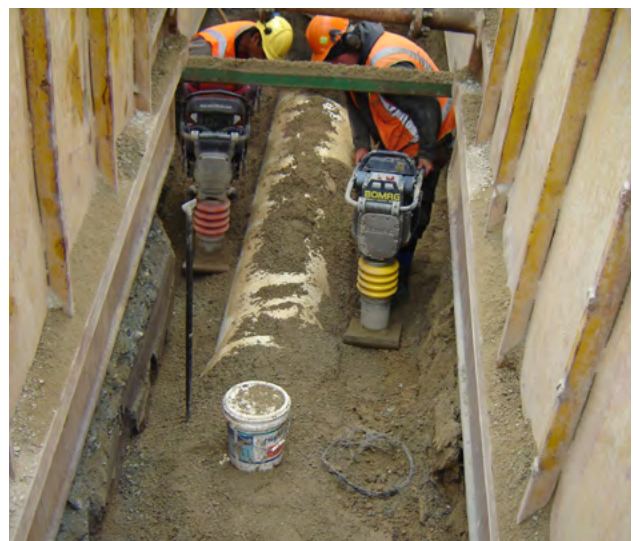
Figure 11.23 - Side compaction of granular bedding and surround material with a trench shield - the side compaction zone is below the shield, directly against the trench wall
