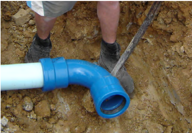
Figure 9.7 - Assemble the fitting onto the PVC-O pipe with a bar. Insert the pipe into the full length of the fitting socket
