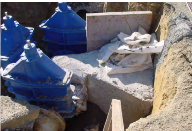
Figure 10.4 - Concrete thrust block supporting a three-way valve assembly, on a PVC transmission water main, Timaru City
