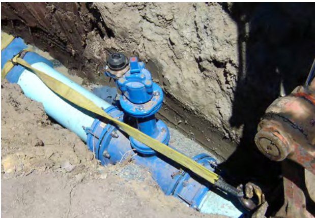
Figure 9.8 - Larger size ductile iron fittings may need extra mechanical help to assemble, such as here, with a lifting strop pulled by the excavator. DN 250 socketed bend being assembled onto a DN 250 Series 2 PN 16 Iplex Apollo® PVC-O watermain near Richmond, Tasman District
