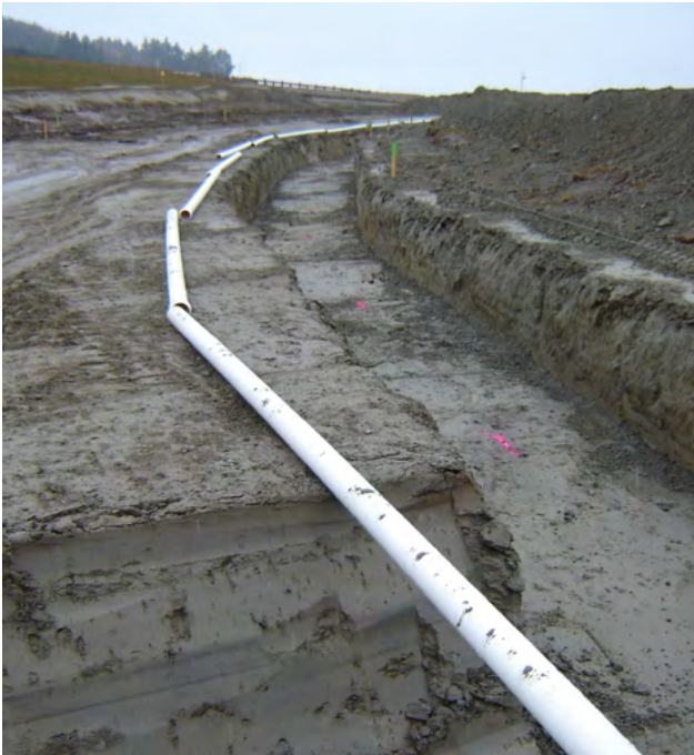
Figure 8.11 - Installing DN 100 S1 PN 12.5 Iplex Apollo® PVC-O pipes in sub-zero winter conditions, for a reticulation Water Main ,Wanaka, Queenstown Lakes District
