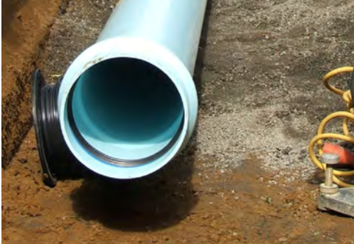
Figure 11.14 - Thoroughly clean seal ring and socket interior. Clear a small space under the socket to ensure the lubricated spigot does not touch the trench or pick up any dirt
