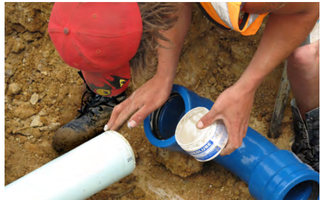
Figure 9.6 - Lubricate the chamfered PVC-O pipe spigot, and fitting seal ring, with Iplex Medlube
