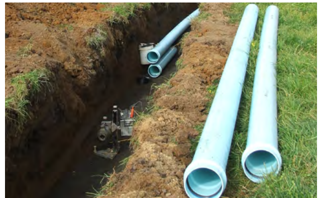
Figure 8.9 - DN 150 S2 PN 16 Iplex Apollo® PVC-O pipe used for a pressure sewer rising main - New Plymouth City, Taranaki
