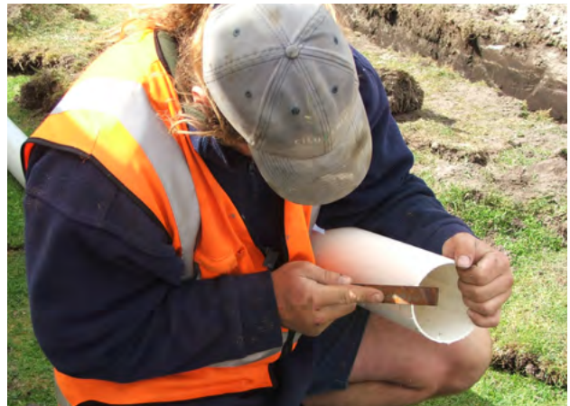
Figure 11.8 - Chamfering pipe with hand file
