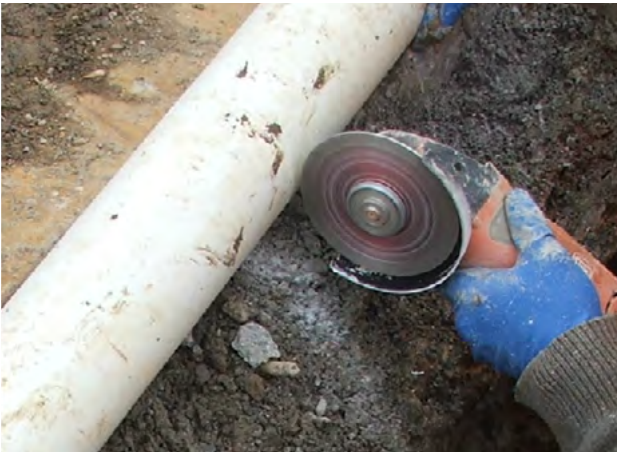
Figure 11.5 - Cutting pipe with power-driven masonry blade
