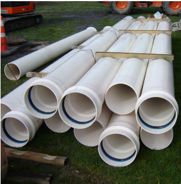
Figure 7.1 - Iplex Apollo® PVC-O DN 200 PN 12.5, pressure sewer main, installed in Charles St, Kaiapoi, October 2010, which endured the February 2011 Christchurch Earthquake sequence, and all following aftershocks undamaged
