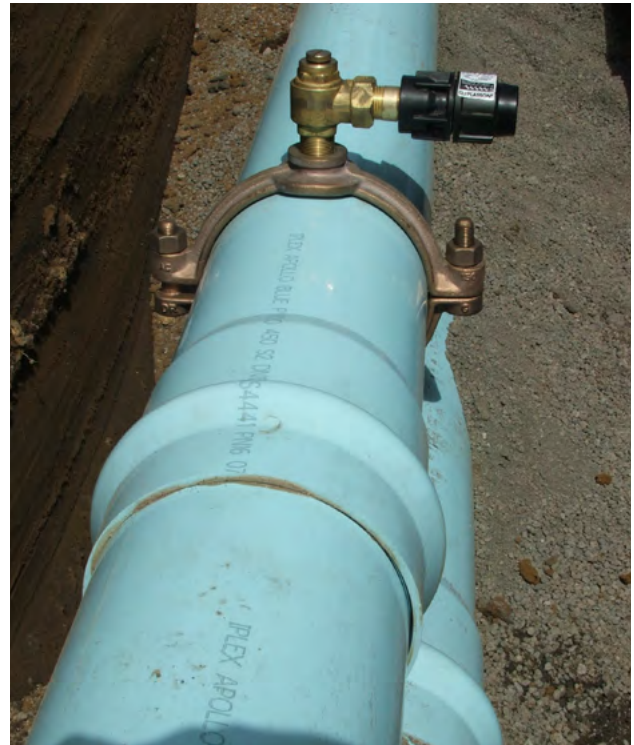
Figure 9.14 - Gunmetal tapping saddle and Under Pressure Tapping ferrule with a Plasson "line 7" male threaded adapter, for an air release point, on a twin, DN 150 Series 2 PN 16 Iplex Apollo® PVC-O pipe, near Oakura, Taranaki district
