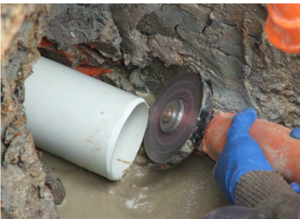
Figure 11.6 - Chamfering pipe with power-driven masonry blade
