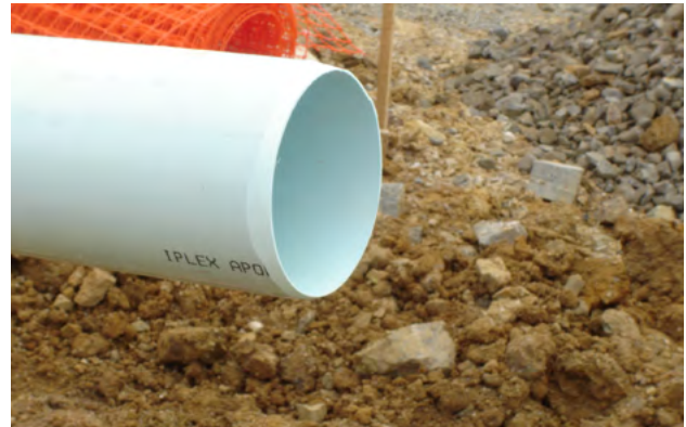
Figure 9.5 - If cutting a pipe on site, cut the pipe square and handchamfer the pipe spigot, similar to a factory produced chamfer
