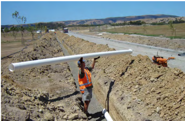
Figure 4.2 - Site handling and installation of Iplex Apollo® PVC-O DN 100 Series 1 PN 12.5, for water distribution in a residential subdivision near Martinborough
