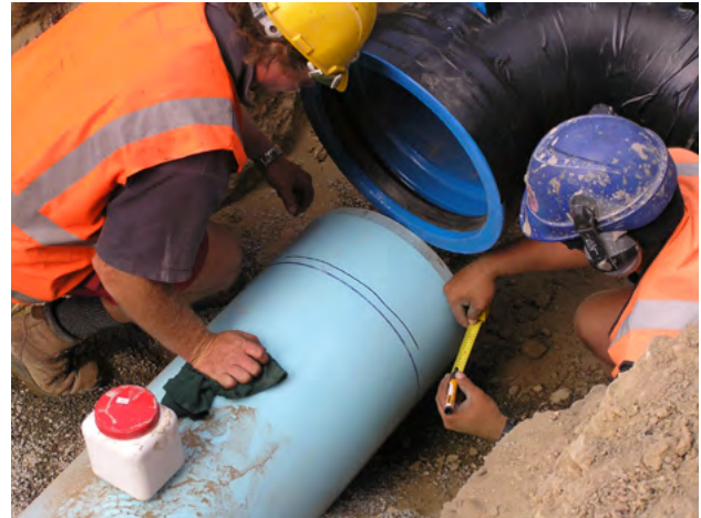
Figure 9.4 - Re position the insertion witness mark on the pipe spigot as needed, to allow for full depth socket insertion
