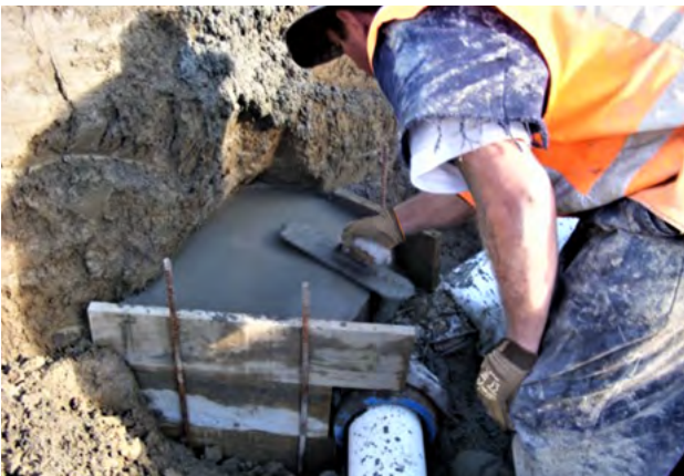
Figure 10.5 - Installing a concrete thrust block on a DN 100, 45 Deg Ductile iron bend, fitted to Iplex Apollo® PVC-O PN 12.5 pipe, Southland District
