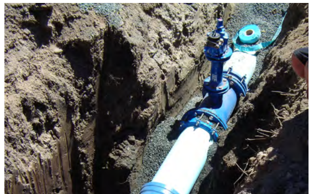
Figure 9.12 - Typical arrangement of "AVK" brand, Universal flange adapters, on a flange branched tee, with hydrant, and hydrant riser, installed onto DN 250 Iplex Apollo® PVC-O pipe, Tasman District
