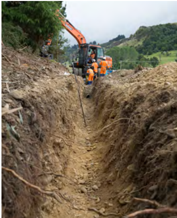
Figure 11.24 - Trench bottom in stoney ground, evenly cut to grade and depth before placing the bedding aggregate. Waitaki District
