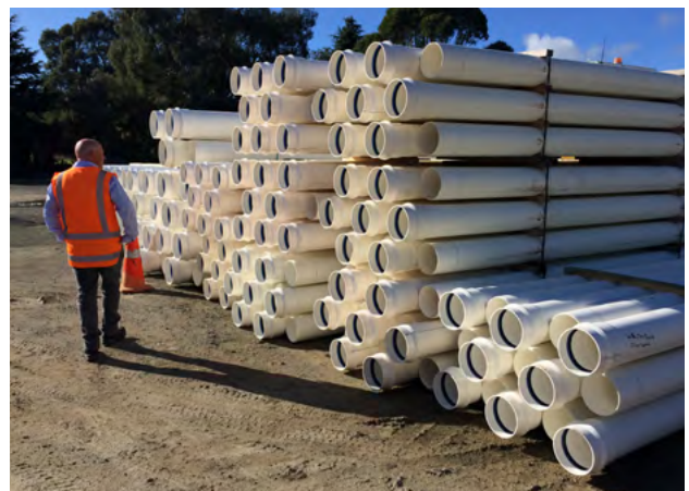
Figure 11.3 - Temporary storage of DN 150 Series 1 Iplex Apollo® PVC-O pipe, in original factory crates on a flat site, near Oamaru, Waitaki District
