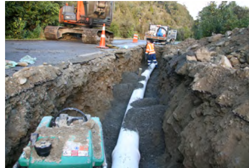
Figure 11.27 - DN 300 Iplex Apollo® PVC-O Series 1 PN 12.5 watermain in 6m lengths, following a curved road alignment, Westland District
