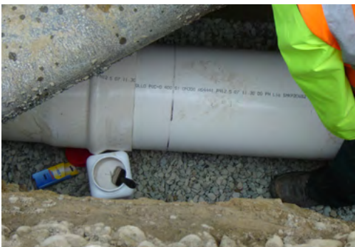
Figure 11.18 - Insert aligned lubricated spigot into socket
