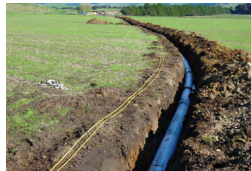
Figure 11.28 - DN 300 Iplex Apollo® PVC-O Series 1 PN 10 watermain in 6m lengths, on a curved alignment, Hawkes Bay District
