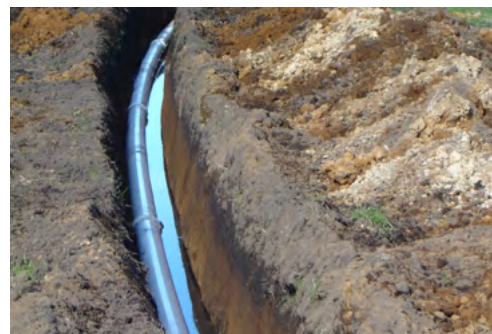
Figure 11.29 - DN 150 Iplex Apollo® PVC-O Series 1 PN 10 watermain, in 6m lengths, on a curved alignment, Hawkes Bay District
