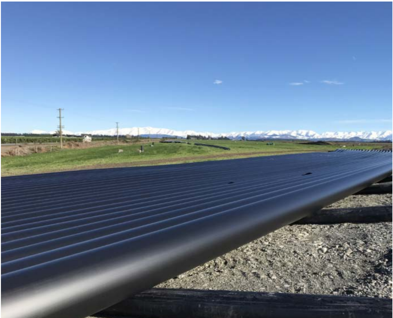
Iplex PE 100 pressure pipe extruded on site in the Central Plains.
