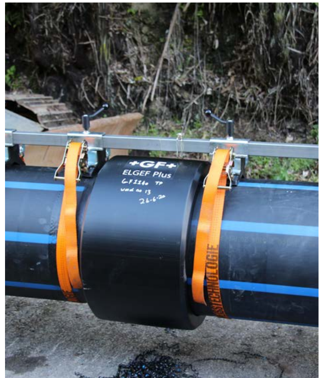
Iplex Poliplex® PE 100 pressure pipe showing electro fusion welding.
