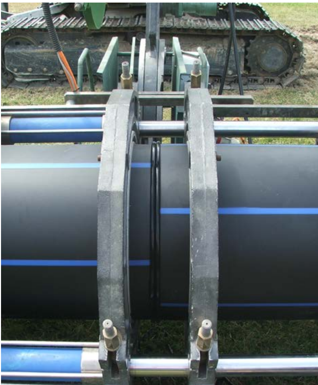
Iplex Poliplex® PE 100 pressure pipe showing butt fusion welding.
