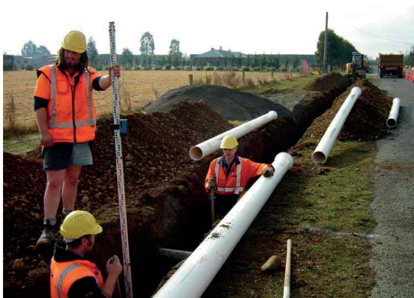
Installation of NOVAKEY™ Series 1 PN 12 pipes, in a road berm near Ashburton, with laser assisted control of the trench depth and grade.
