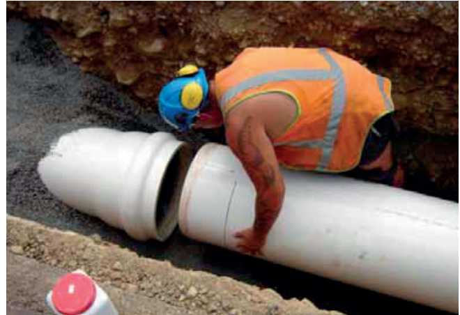
Joint assembly on NOVAKEY™ DN 450 PN12 watermain under a sealed main highway.
