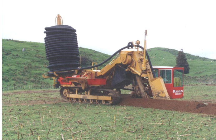
Trenched Installation of 110mm Iplex NOVAFLO subsoil drainage pipe, in 450m rolls, using laser-guided gradient control
