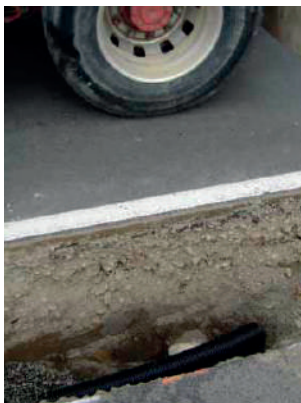
Iplex NEXUSFLO interceptor drain installation under the berm of an arterial commercial/industrial roading environment, Tremaine Avenue, Palmerston North City.
