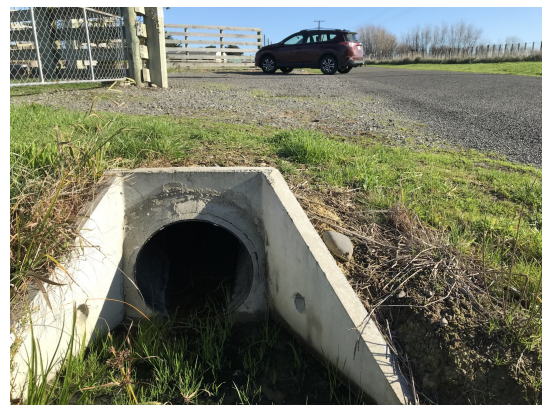
Application of Iplex NEXUS™ Culvert under a farm vehicle-access to stock loading yards, with "wing walls" to protect the bedding and backfill from erosion, around the pipe entry and exit positions.
