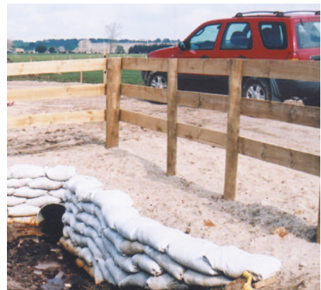
Application of Iplex NEXUS™ Culvert under a farm vehicle-access to stock loading yards, with "wing walls" to protect the bedding and backfill from erosion, around the pipe entry and exit positions.
