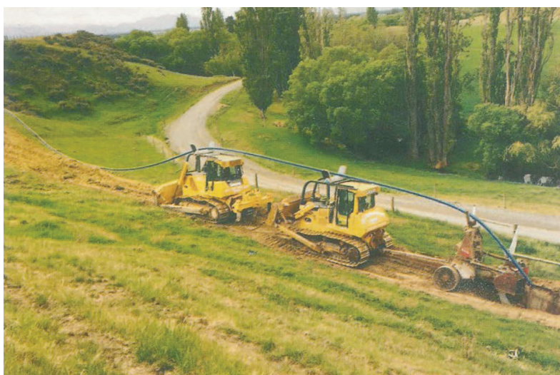
Mole Plough installation of Iplex Rural PE pipes.
