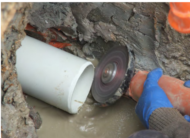
Figure 6.6 - Chamfering pipe with power-driven masonry blade
