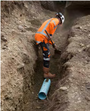
Figure 6.24 - Placing the selected size imported bedding aggregate, fully surrounding the pipe, Waitaki District
