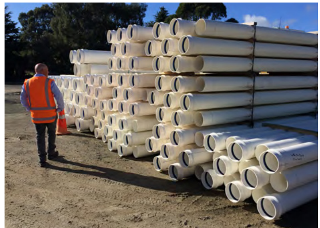
Figure 6.3 - Temporary storage of DN150 Series 1 Iplex PVC pipe, in original factory crates on a flat site, near Oamaru, Waitaki District
