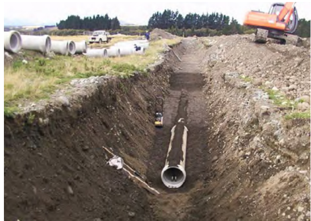
Iplex® PVC-U DN450 sewer main installed in Te Anau 2001, to replace a earthquake damaged concrete pipeline, and which has endured all earthquakes in the area since, undamaged.
