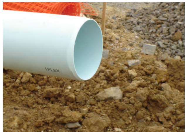
Figure 6.9 - Hand- chamfered Iplex PVC pipe spigot
