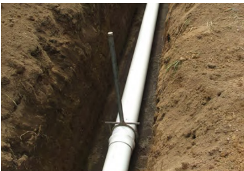
Figure 6.19 - Positioning of pipe jointing fork
