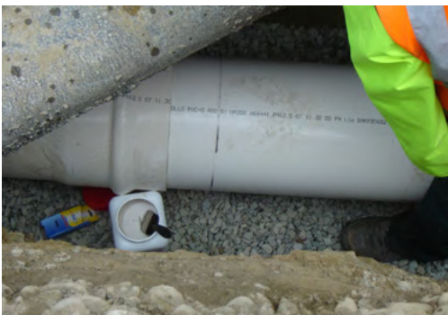
Figure 6.17 - Insert aligned lubricated spigot into socket
