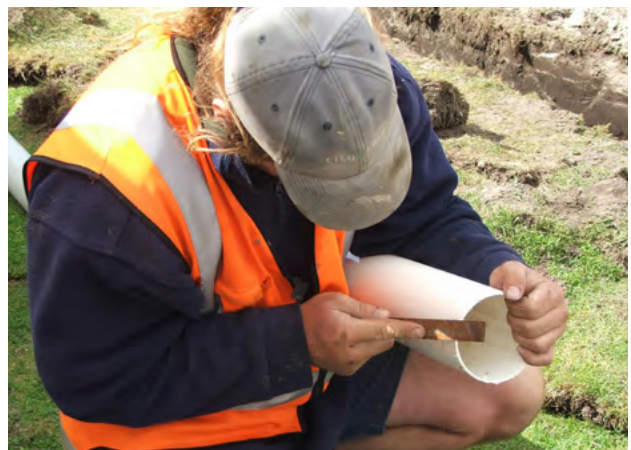
Figure 6.8 - Chamfering pipe with hand file
