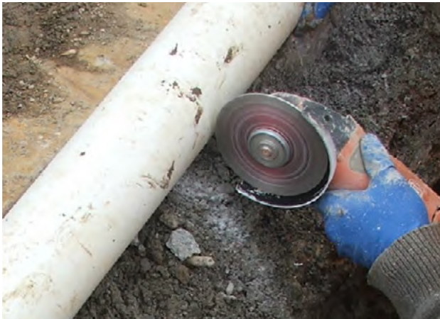
Figure 6.5 - Cutting pipe with power-driven masonry blade
