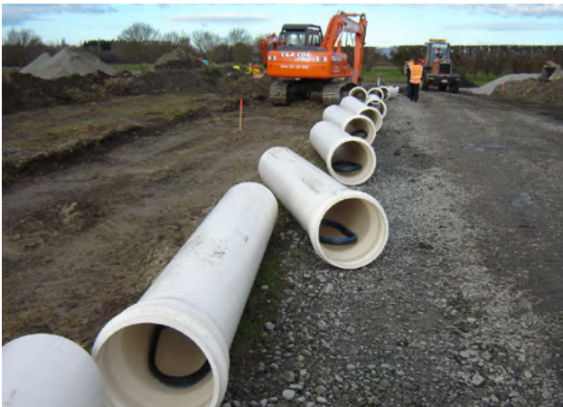
Iplex Novakey® DN450 PVC-U pressure sewer rising main, laid near Belfast, Christchurch in 2005, which endured the 2011 Canterbury earthquake sequences, undamaged.
