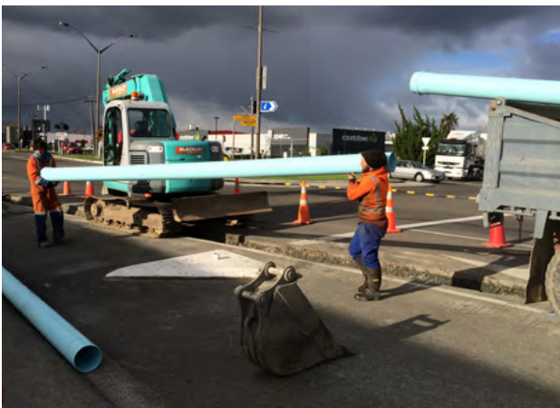
Figure 6.1 - Handling and unloading of DN150 Iplex PVC pipe, preventing abrasion damage from the truck deck or by impacting the road surface. - Feilding, Manawatu District
