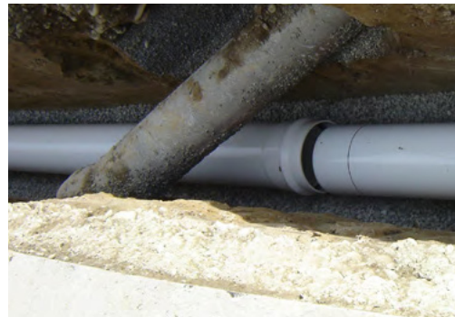
Figure 6.16 - Align the lubricated spigot with the socket mouth
