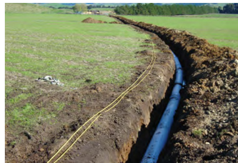
Figure 6.27 - DN300 Iplex PVC watermain, in 6m lengths, on a curved alignment, Hawkes Bay District
