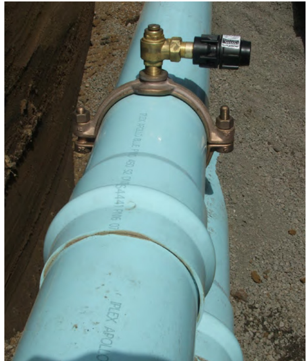
Figure 3.13 - Gunmetal tapping saddle and Under Pressure Tapping ferrule with a male threaded adapter, for an air release point, on a twin, DN150 Series 2 PN16 Iplex® PVC pipe, near Oakura, Taranaki District
