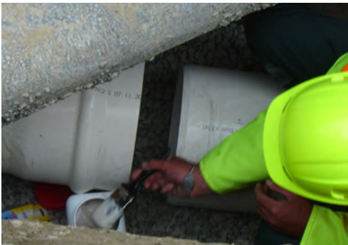
Figure 6.15 - Apply Medlube lubricant to both the seal and the spigot with a clean brush
