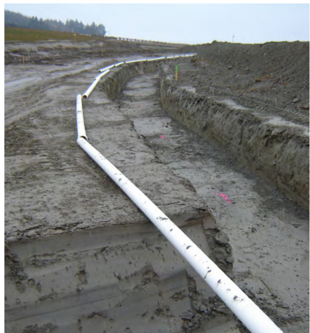
Figure 4.8 - Installing DN100 S1 PN12.5 Iplex PVC pipes in winter conditions, for a reticulation Water Main, Wanaka, Queenstown Lakes District
