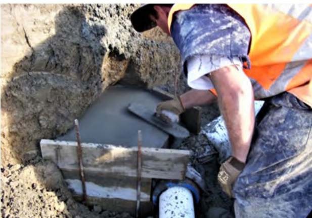
Figure 5.5 - Installing a concrete thrust block on a DN100, 45 Deg Ductile iron bend, fitted to Iplex PVC PN12.5 pipe, Southland District
