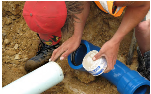
Figure 3.5 - Lubricate the chamfered PVC pipe spigot, and fitting seal ring, with Iplex® Medlube
