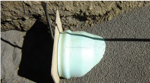
Figure 6.12 - Protect the clean socket from entry of dirt and grit, before joint assembly
