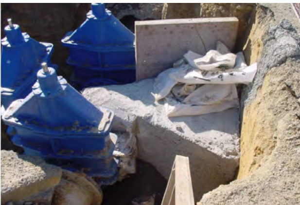
Figure 5.4 - Concrete thrust block supporting a three-way valve assembly, on a PVC transmission water main, Timaru City
