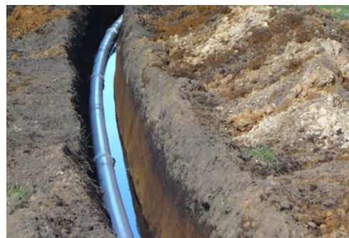
Figure 6.28 - DN150 Iplex PVC watermain, in 6m lengths, on a curved alignment, Hawkes Bay District
