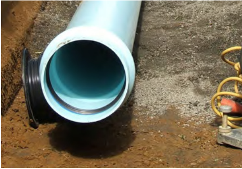
Figure 6.13 - Thoroughly clean seal ring and socket interior. Clear a small space under the socket to ensure the lubricated spigot does not touch the trench or pick up any dirt
