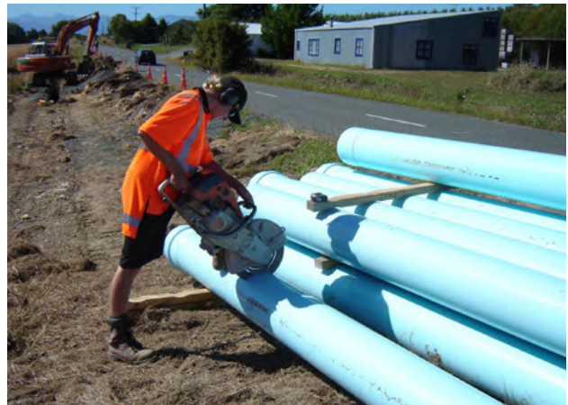
Figure 6.7 - Cutting pipe with power-driven masonry blade
