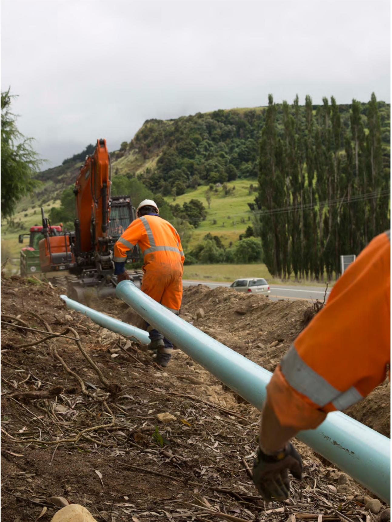
Iplex PVC Series 2 pressure transmission water main installation, Waitaki District.
