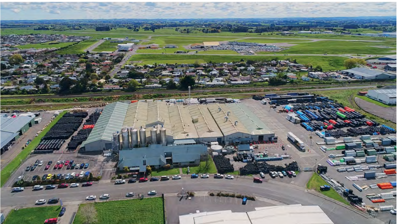
Iplex Pipelines manufacturing plant and distribution hub in Palmerston North, New Zealand.
