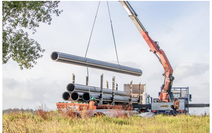
First delivery of Iplex DN710 PE pipe arriving at Schnapper Rock.
