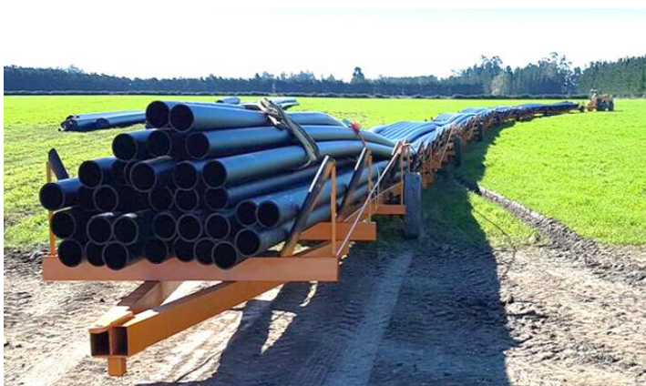
Wheel dollies with pipe loaded ready for transportation
