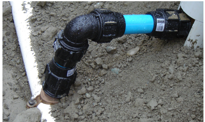
BlueLine pipe and compression fittings used for a water service connection off a PVC-O main to a residential property near Wanaka.
