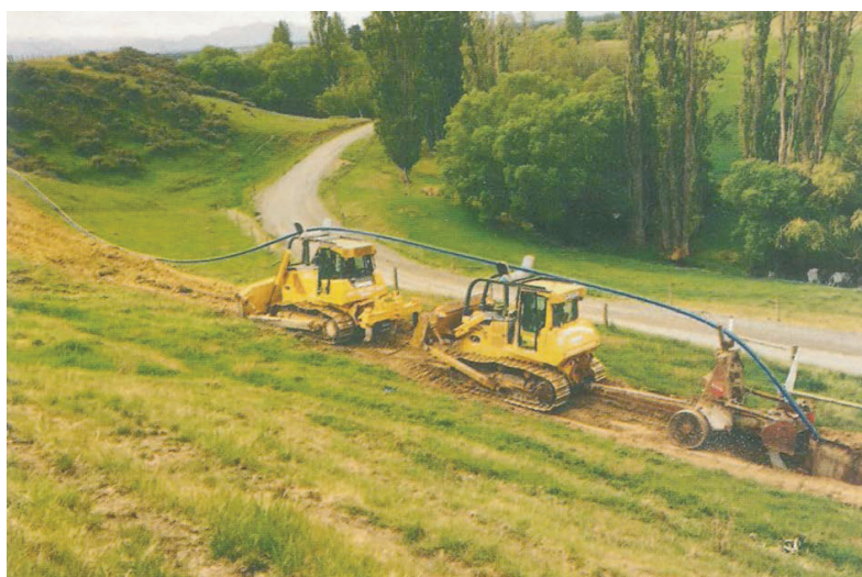
Mole Plough installation of Iplex Blackline pipes.
