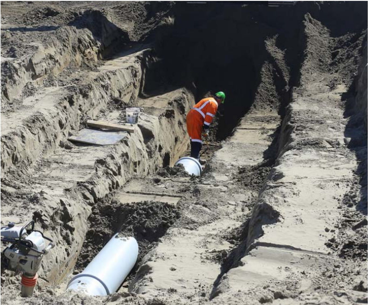
Iplex Superstorm® being installed on the Mackays to Peka Peka Expressway project, Kapiti Coast
