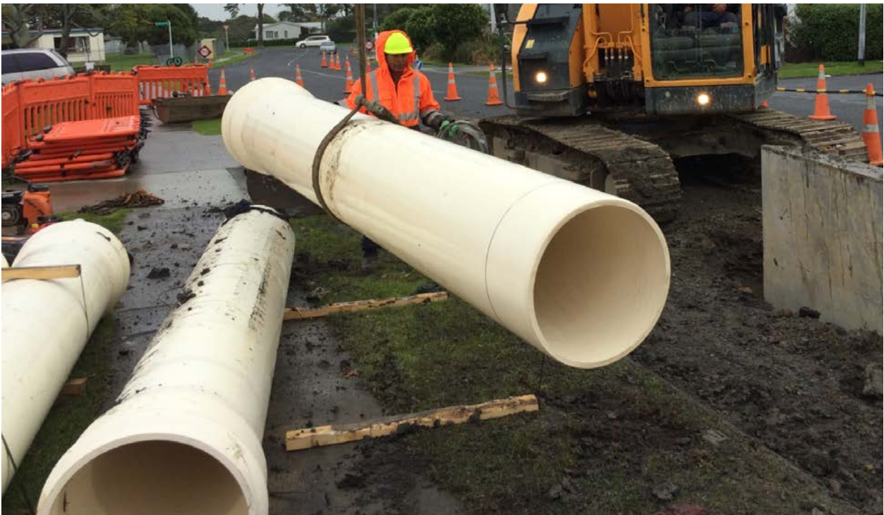
Installation of DN 600 Iplex Novadrain® PVC-U pipe for trunk sewer in Mangere, Auckland.
