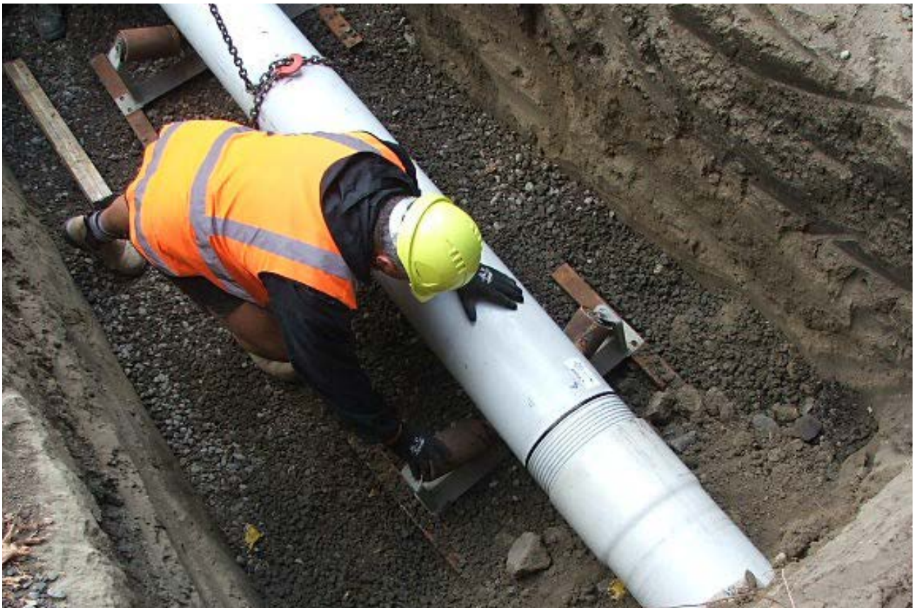
Iplex Restrain® being installed using static pipe bursting method.
