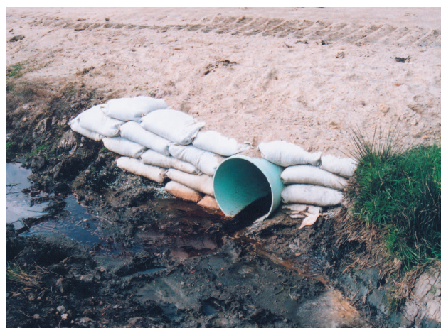
Typical location of Iplex Farmtuff PVC culvert under a farm vehicle-access raceway, with banded support walls to protect the bedding and backfill fill from erosion, around the pipe entry and exit positions.
