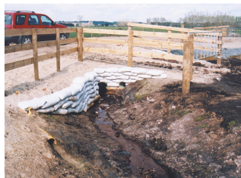
Typical location of Iplex Farmtuff PVC culvert under a farm vehicle-access raceway, with banded support walls to protect the fill from erosion, around the pipe entry and exit positions.
