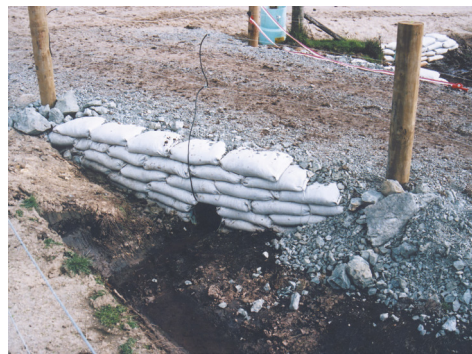
Typical location of Iplex Farmtuff PVC culvert under a farm vehicle-access raceway, with banded support walls to protect the fill from erosion, around the pipe entry and exit positions.
