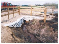
Typical location of Iplex Farmtuff PVC culvert under a farm vehicle access way, with bunded support walls to protect the fill from erosion, around the pipe entry and exit positions.
