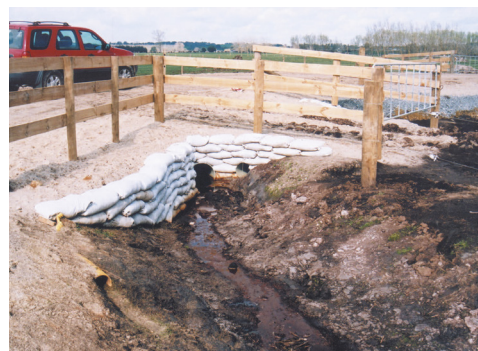
Typical location of Iplex Farmtuff PVC culvert under a farm vehicle-access raceway, with bundled support walls to protect the fill from erosion, around the pipe entry and exit positions.
