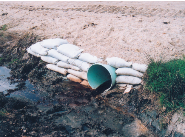
Typical location of Iplex Farmtuff PVC culvert under a farm vehicle-access raceway, with bunded support walls to protect the bedding and backfill fill from erosion, around the pipe entry and exit positions.
