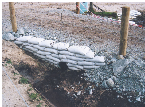
Typical location of Iplex Farmtuff PVC culvert under a farm vehicle-access raceway, with bundled support walls to protect the fill from erosion, around the pipe entry and exit positions.
