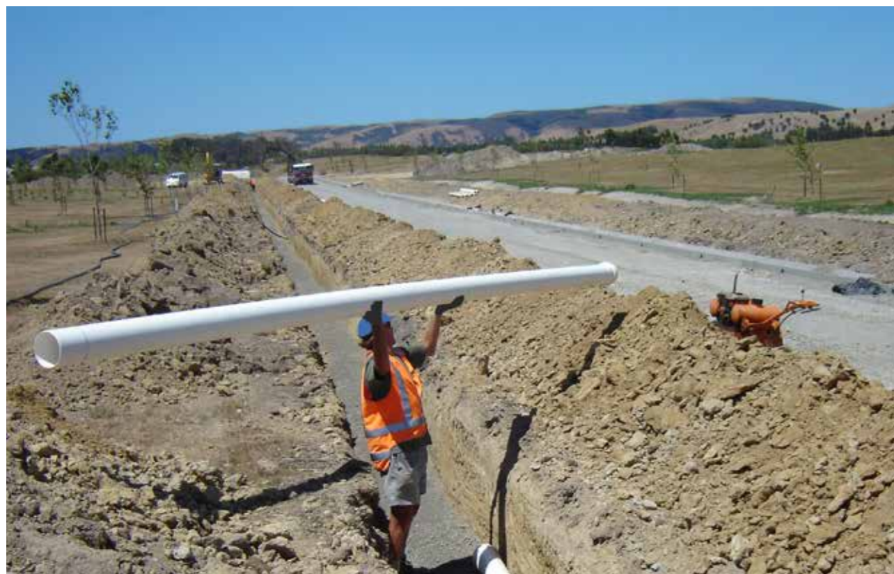
Image 1. Iplex PVC-O Pressure Pipe being installed
