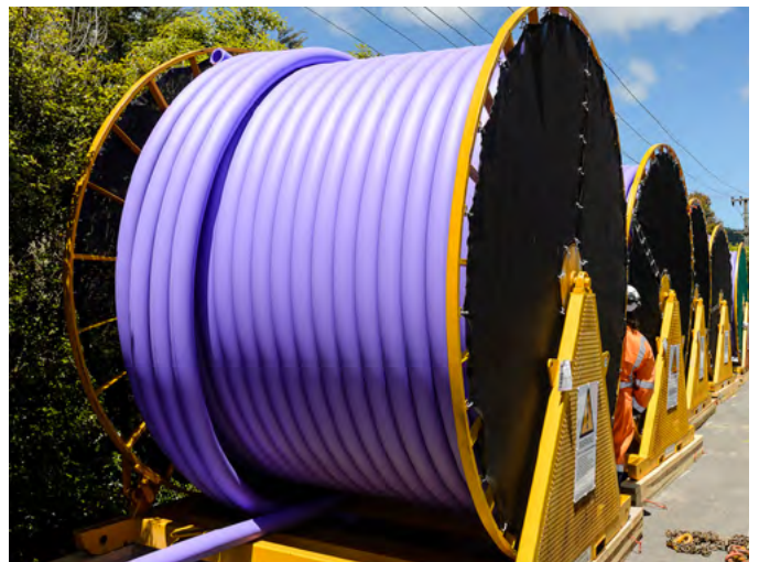
Drum Coils – DN 110 PE Communications duct SDR17
