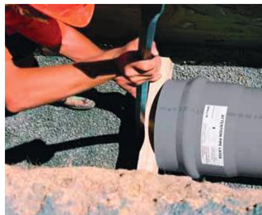
Figure 14 - Push joint home until witness mark remains just visible
