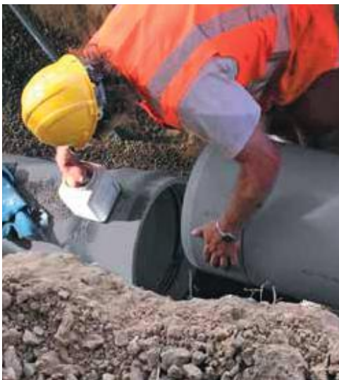
Figure 17 - Lubricate seal and pipe spigot
