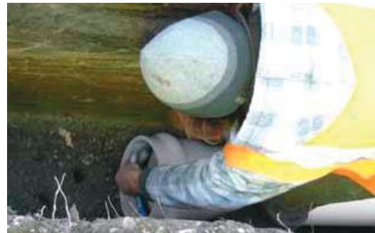
Figure 12 - Apply lubricant to seal with a brush
