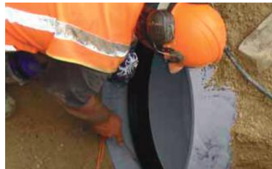
Figure 10 - Clean pipe seal within the socket
