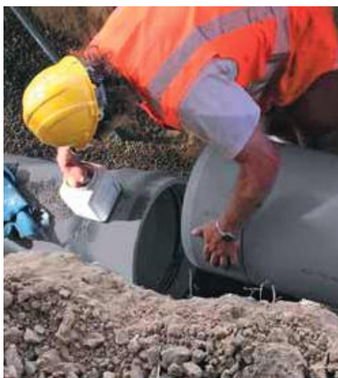
Figure 17 - Lubricate seal and pipe spigot
