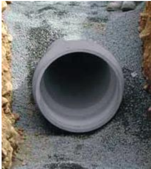
Figure 15 - Thoroughly clean and dry empty pipe socket
