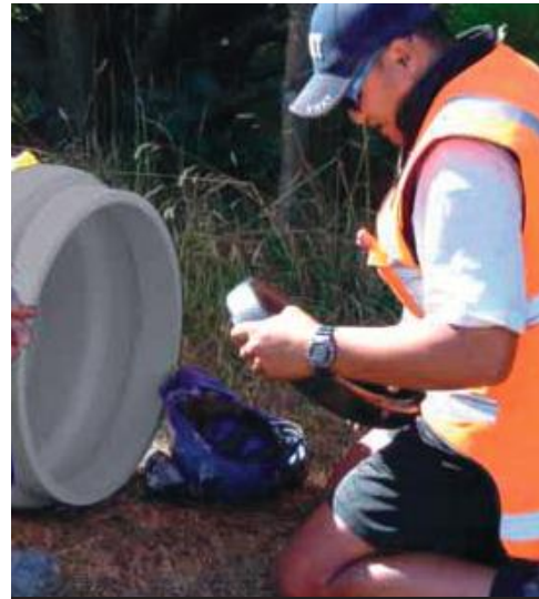
Figure 16 - Fold seal ring and insert into pipe socket
