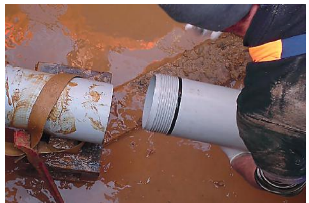
Iplex Restrain™ threaded spigot and socket pipe joint with axial end load restraint capability.
