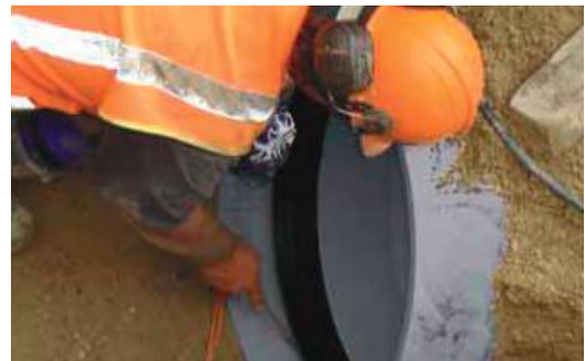
Figure 10 - Clean pipe seal within the socket
