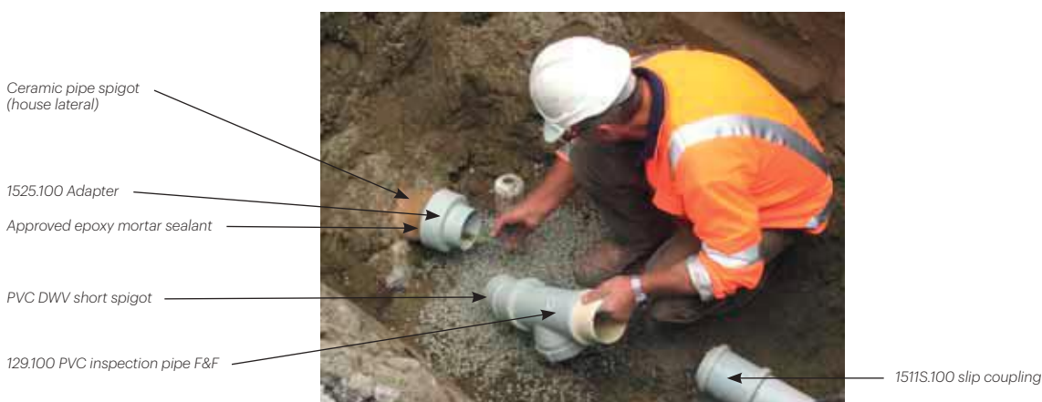
Figure 34 Ceramic Socket to PVC Adapter typical installation
