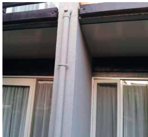
Figure 1: Exposed PVC pipe protected from weathering with UV resistant water-based paint, Dunedin City.
