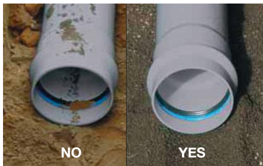
Figure 9 - Thoroughly clean pipe socket and locked in place seal
