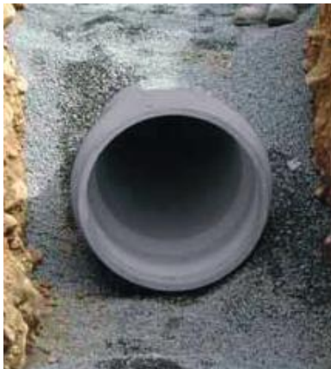
Figure 15 - Thoroughly clean and dry empty pipe socket
