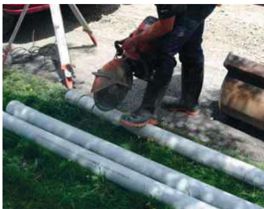
Figure 6 - Cutting pipe with power-driven masonry blade
